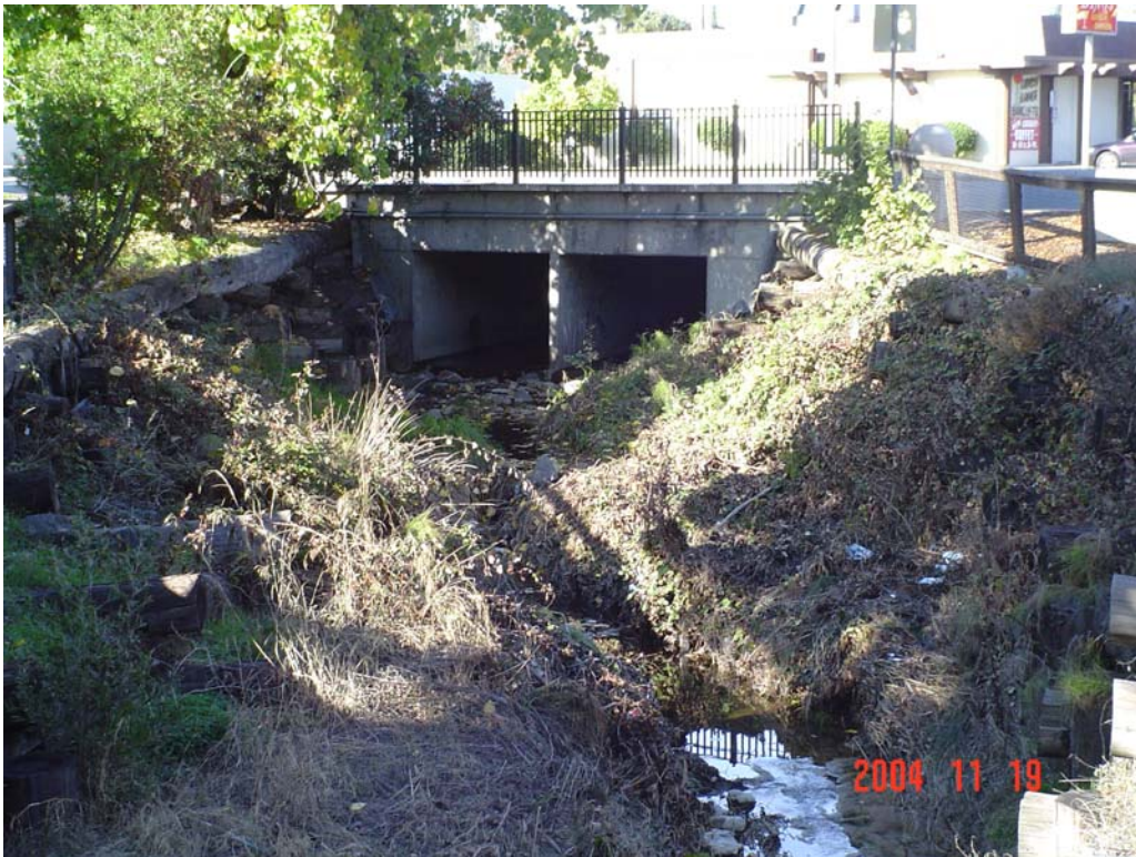
Plate 2: Looking upstream towards the Castro Valley Boulevard
