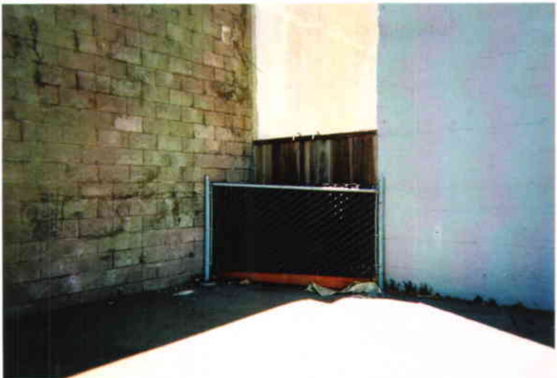
Photo 4: Small Enclosure; Southwest corner of parking lot
