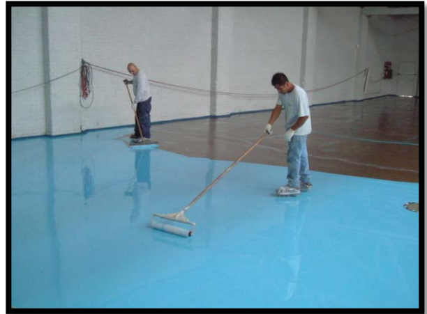
Application of Retro-Coat SEALANT to a 20 mil total thickness
