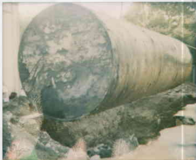
10,000 gal UST being lifted from pit
