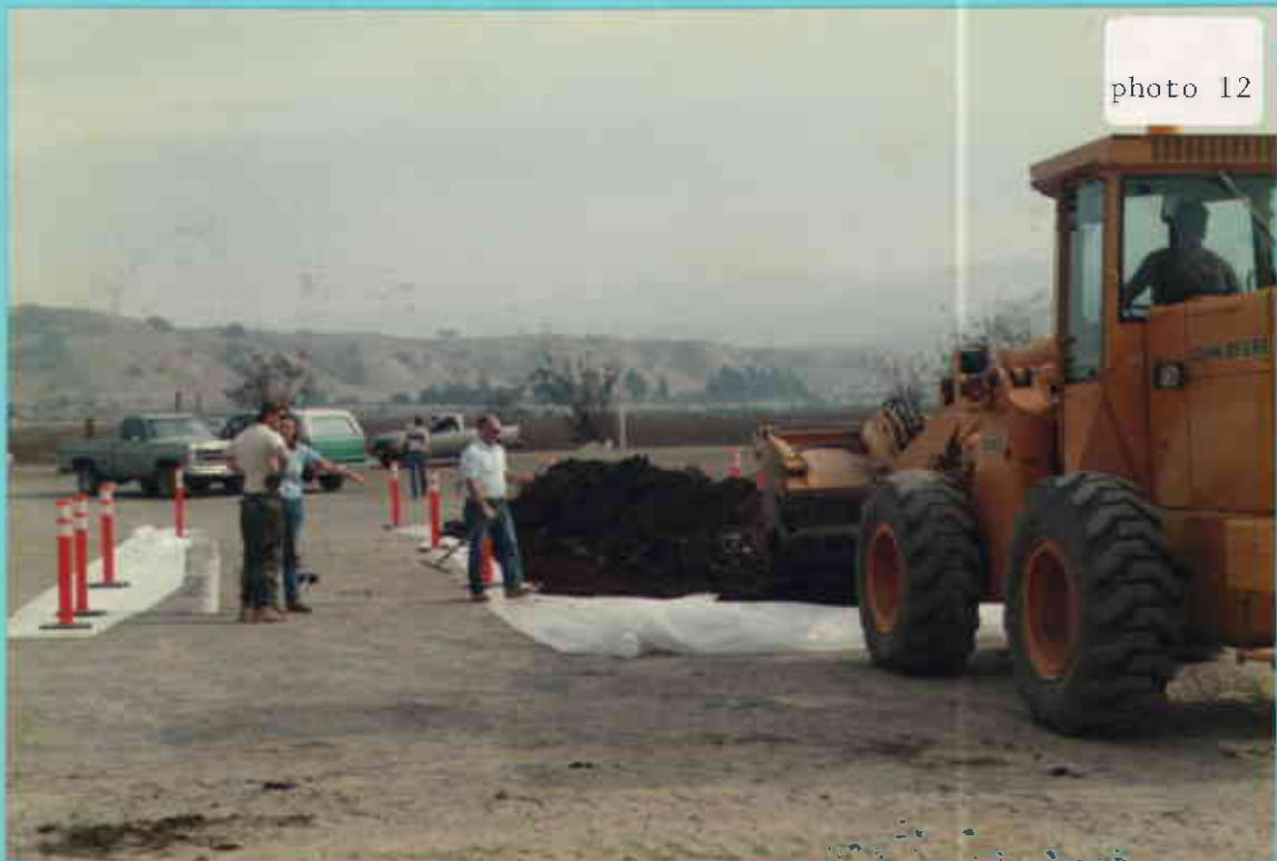
Photo 12. Contaminated soil being placed on visqueen for bio-remediation process on-site.
