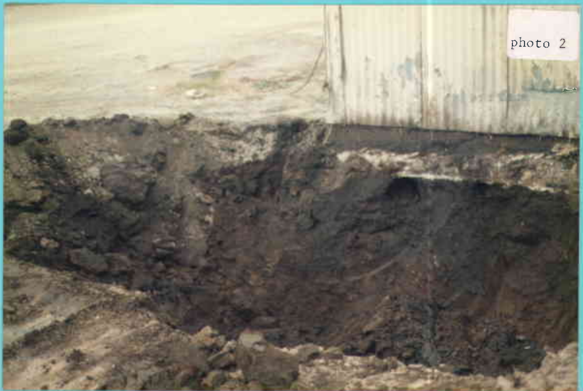
Photo 2. Photo showing contaminated soil (dark gray) directly below the storage shed.
