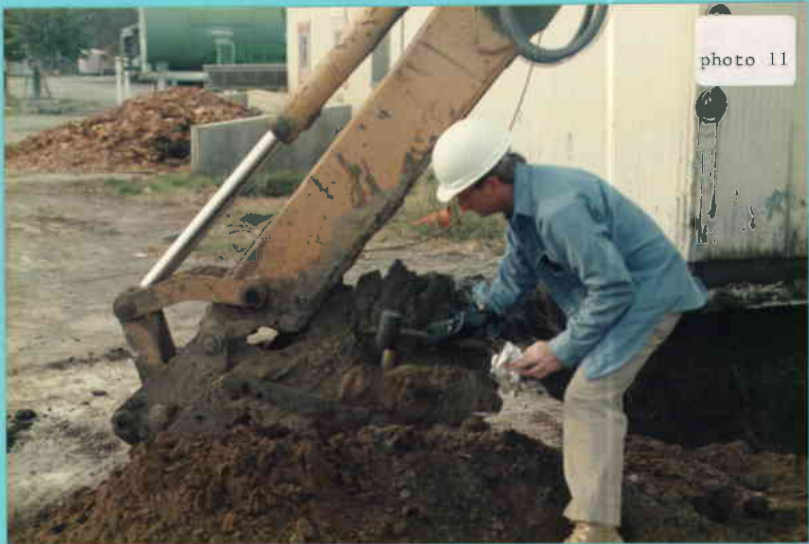
Photo 11. SFDPH engineer taking conformation soil sample, Sunol No.4, in brass tube from soil in south end of excavation.
