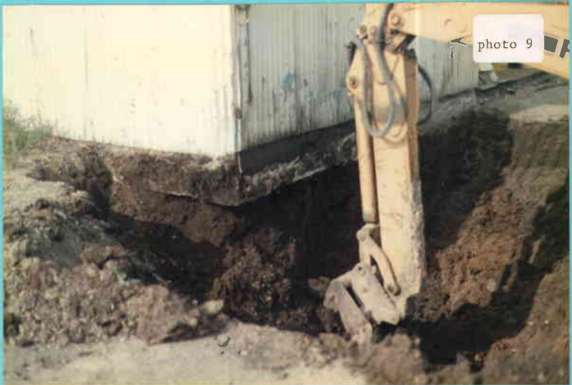
Photo 9. Excavating in area where sample Sunol No.4 was taken.
