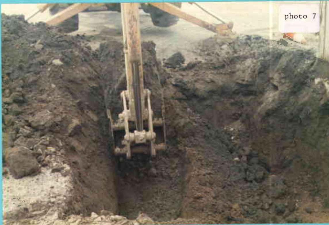
Photo 7. Excavation of contaminated soils near center of pit.
