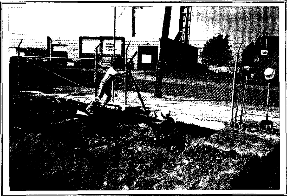
FIGURE 4A - Removal of concrete, soil overburden material, pump dispensers and associated product lines.
