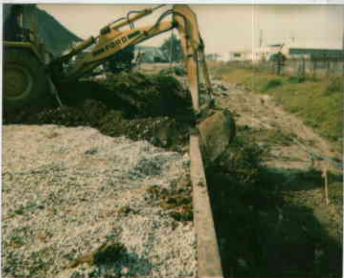
SPD-4051 4015 Hall's St Emeryville 4/1/83 Backland - retaining wall removal.
