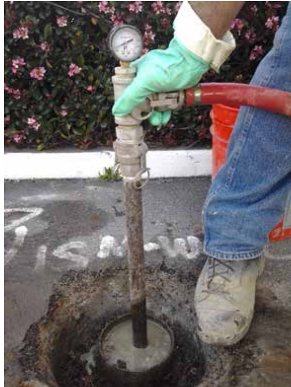
Pressure grouting MW-1.
