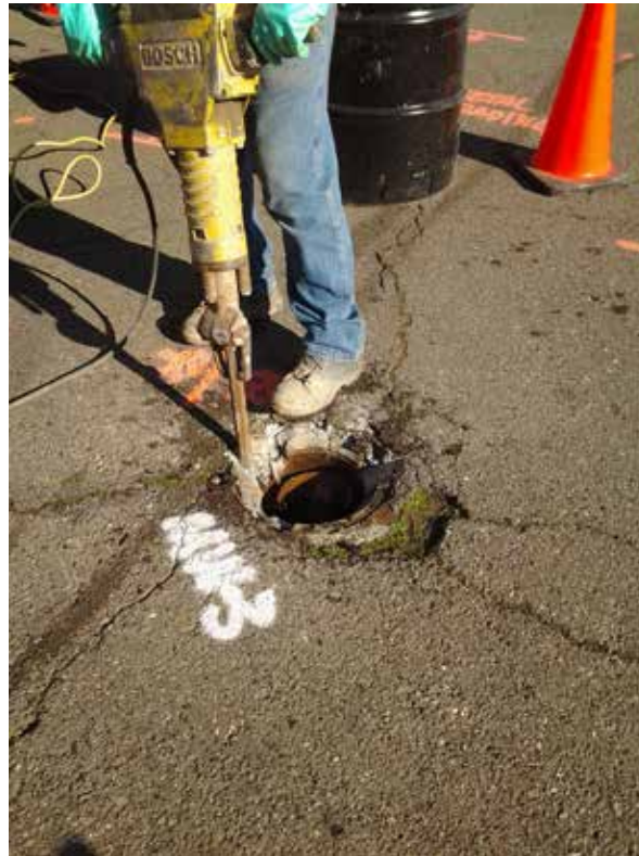
Jack hammering and removing MW-3 well box.
