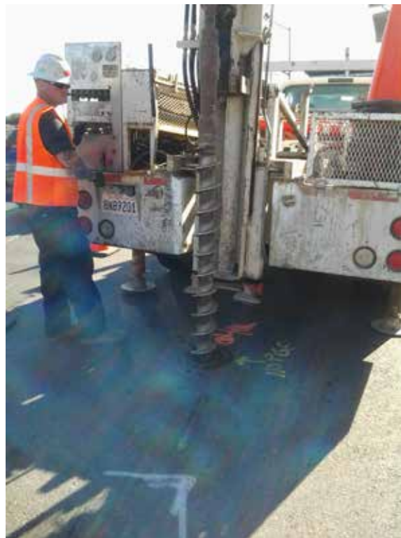
Overdrilling top 5 feet of MW-6.
