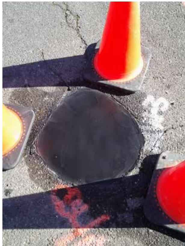
MW-3 surface completion.
