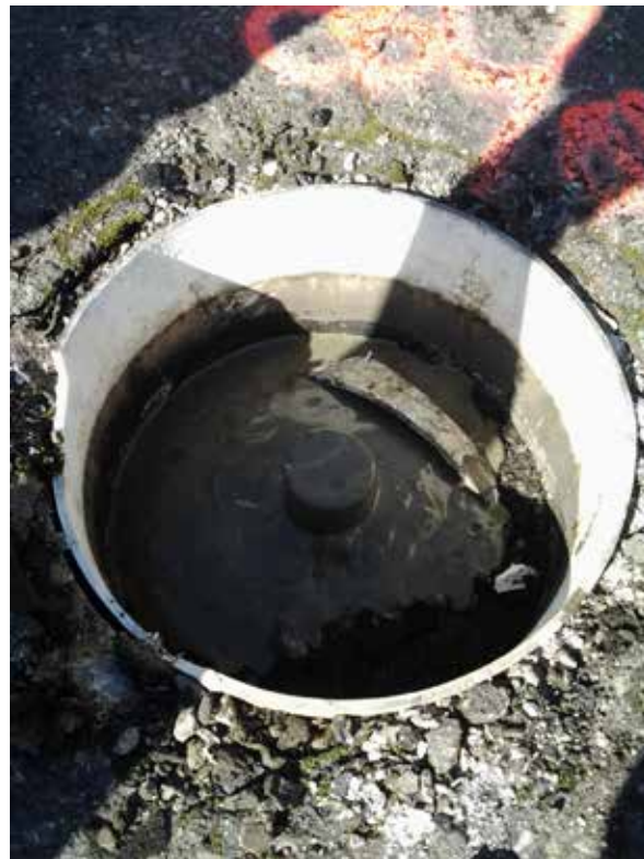
MW-4 grouted to surface.
