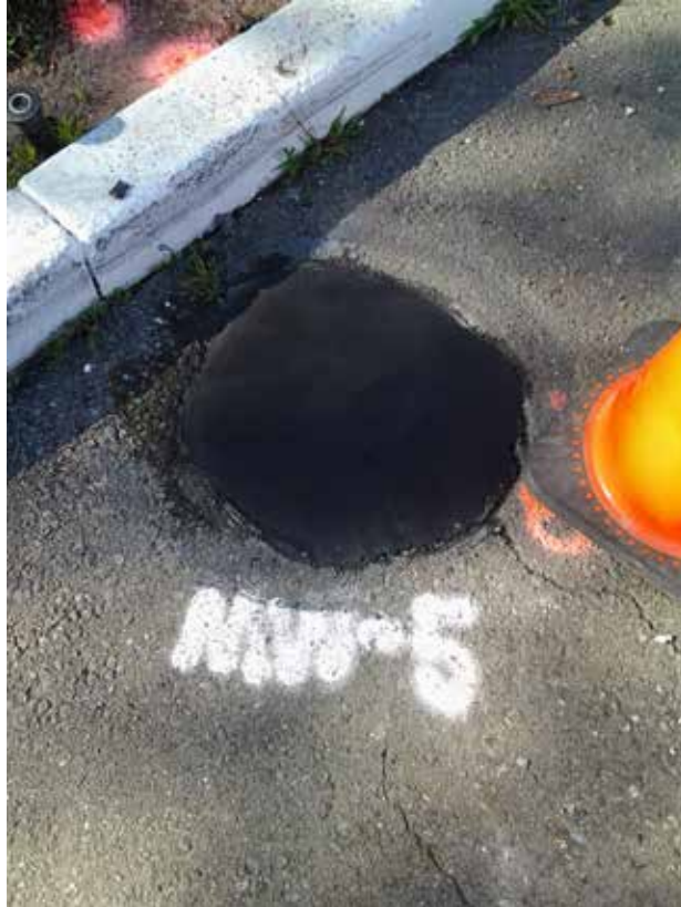
MW-5 surface completion.
