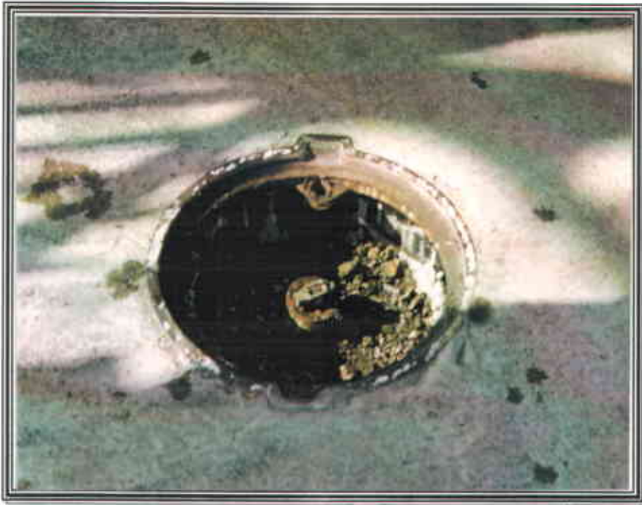
Photo No. 1- Typical monitoring well prior to abandonment.
