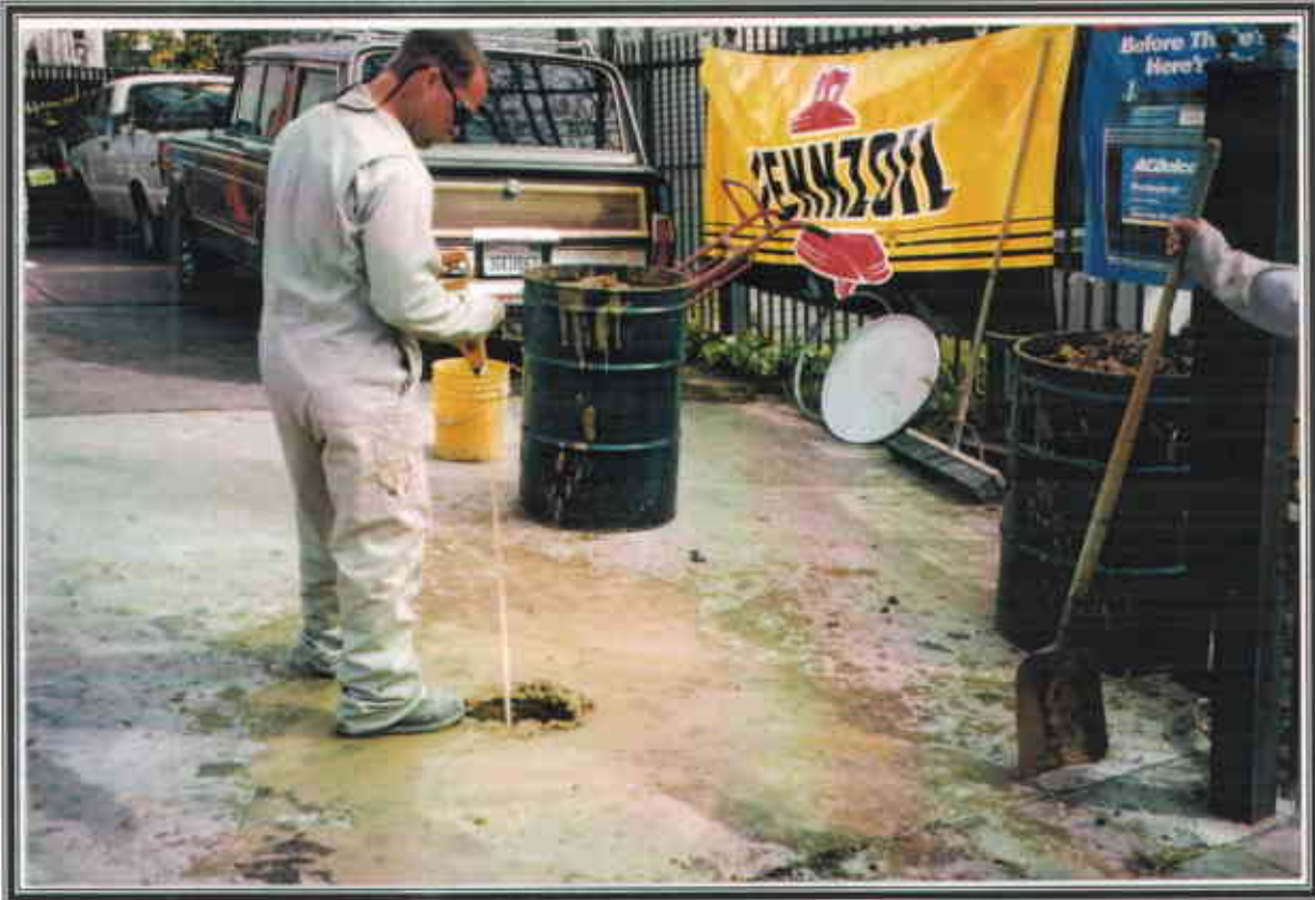
Photo No. 3- Monitoring well after removal of casing and annular materials.
