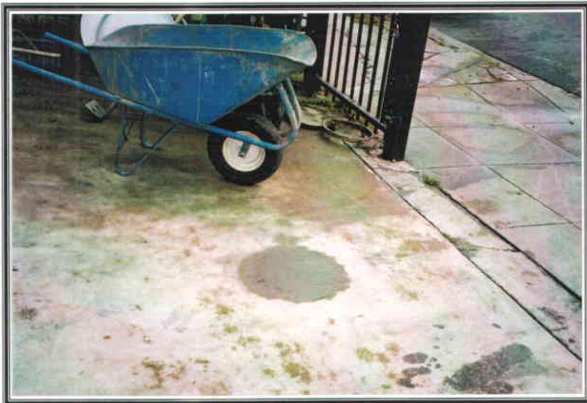
Photo No. 4- Completed abandonment of monitoring well and concrete seal.
