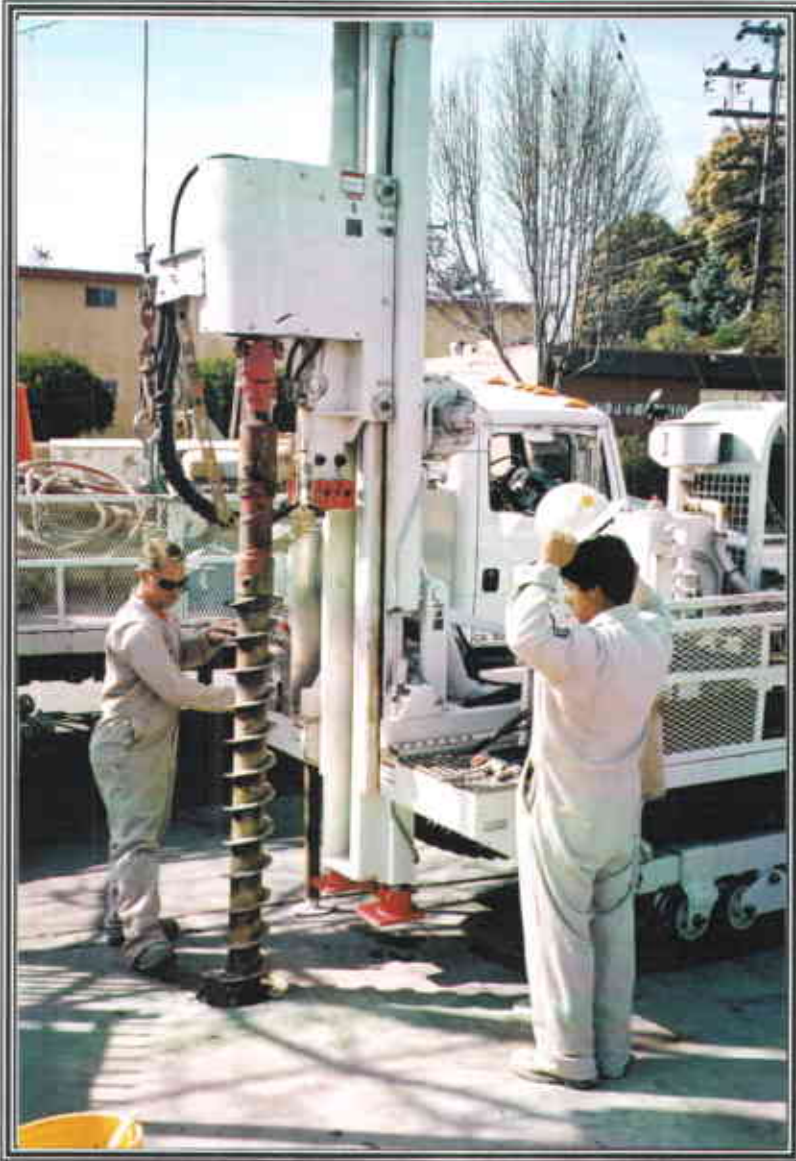
Photo No.2- Overdrilling for removal of casing and annular materials.
