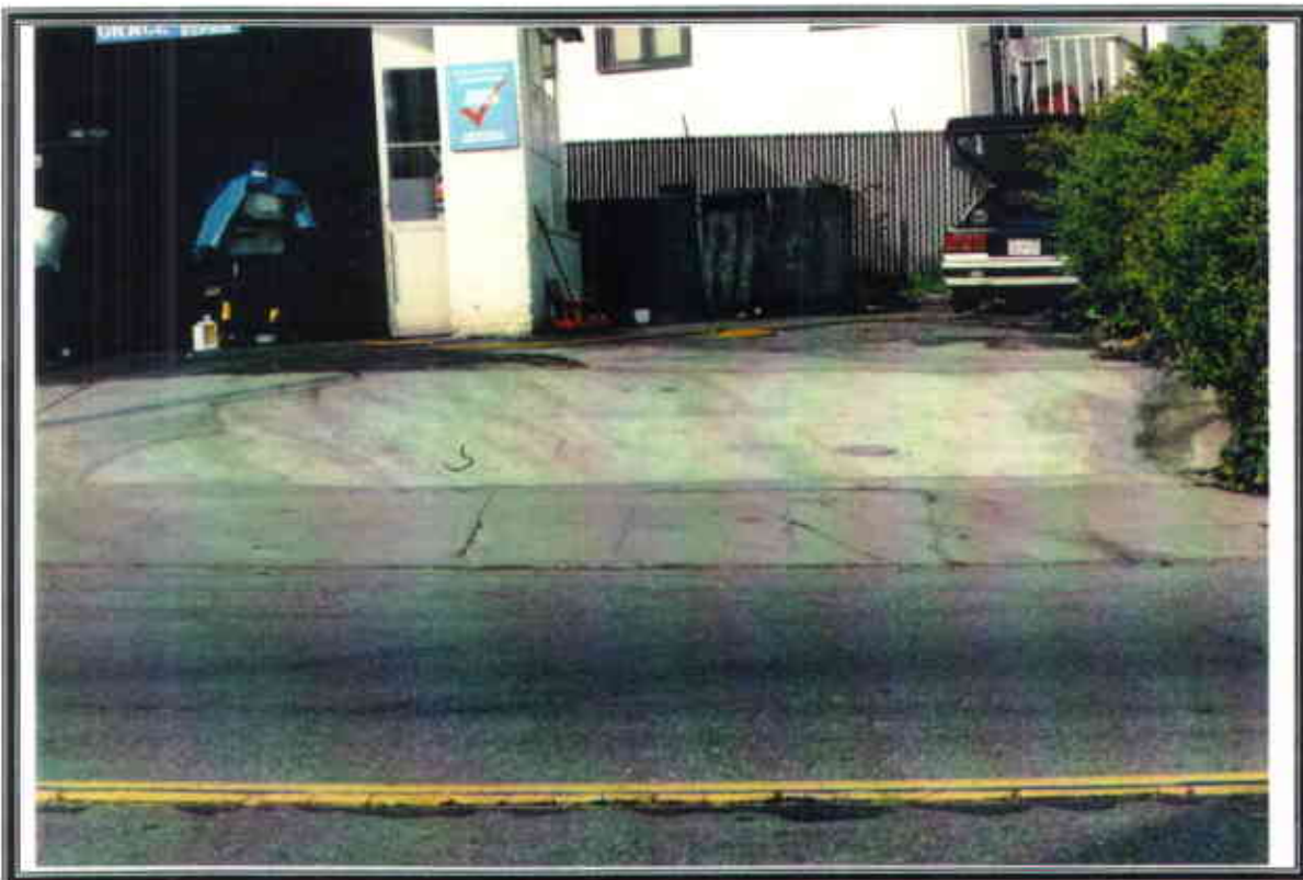
Photo No. 10- Completed work area near monitoring well MW-B1
