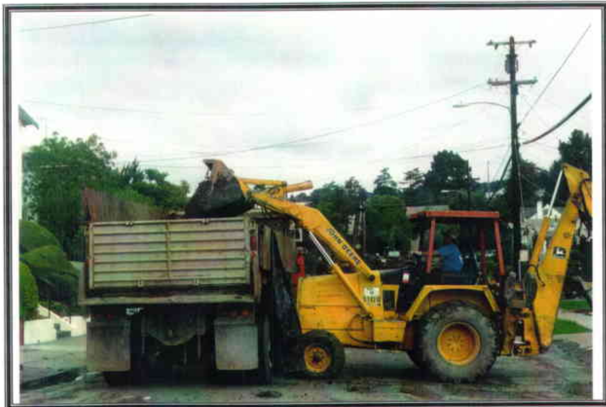
Photo No. 4- Loading contaminated soil into trucks for disposal
