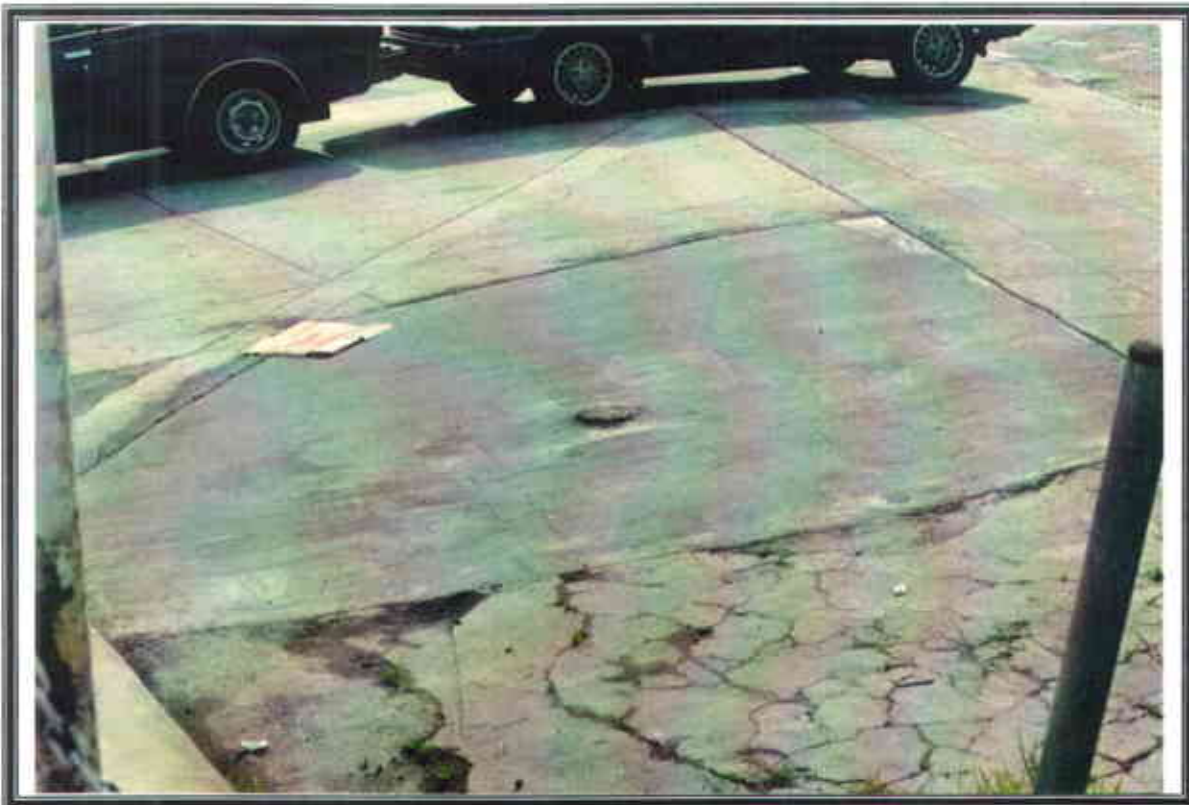
Photo No. 9- Completed work area near monitoring well MW-B3
