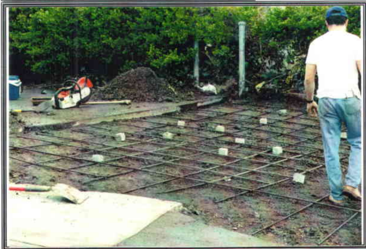
Photo No. 6- Reinforcing bars for concrete resurfacing over the fill
