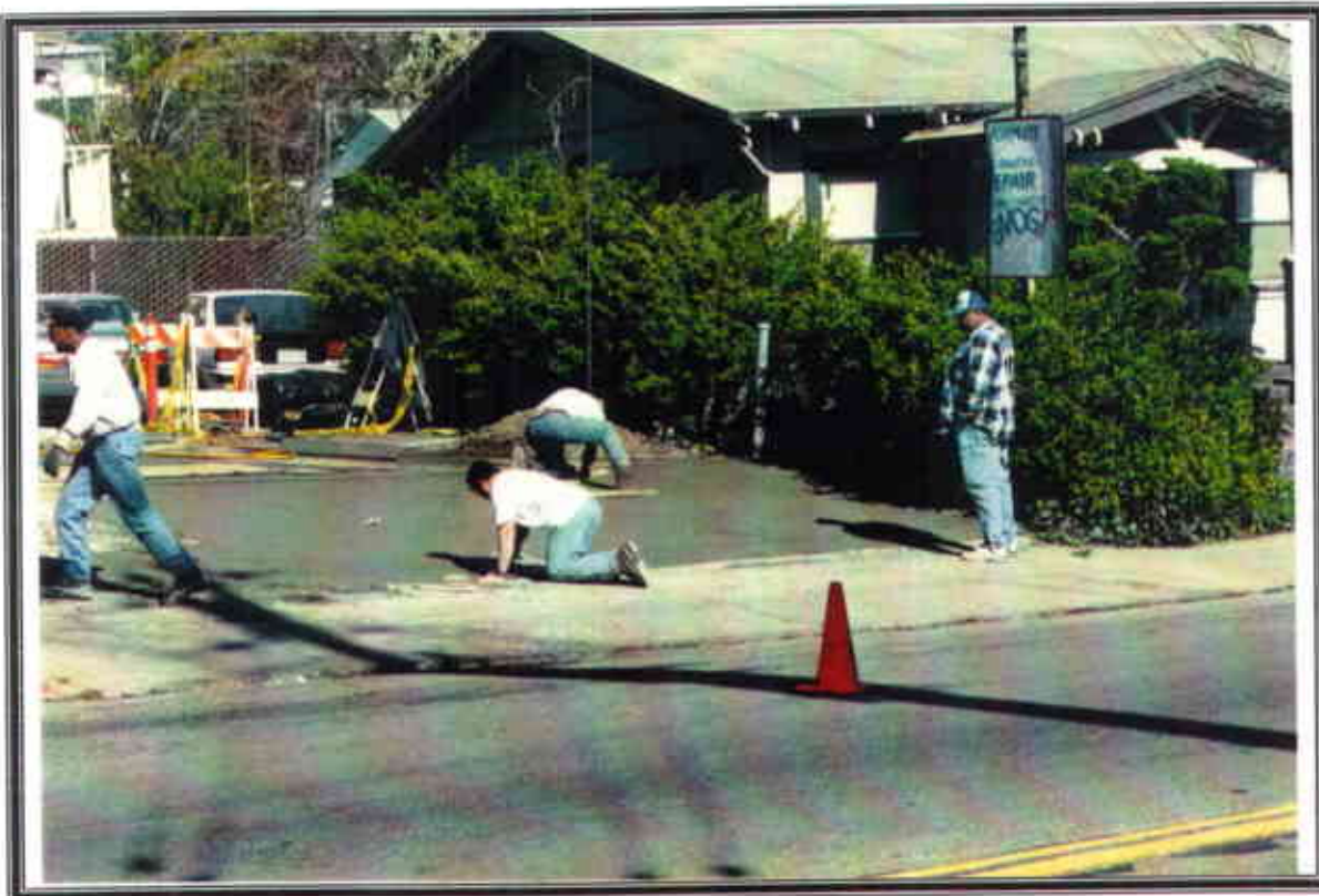
Photo No. 8- Resurfacing with concrete
