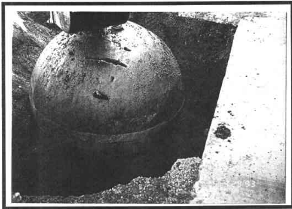
Bulk oil tank removal process. Tank was removed basically intact
