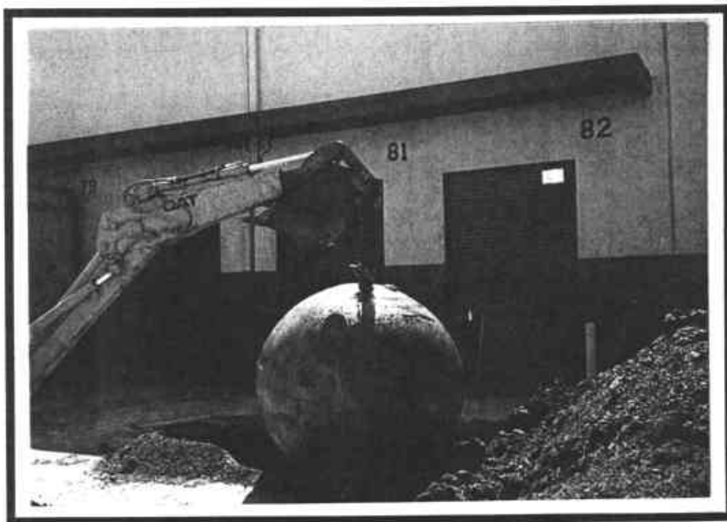
Bulk oil tank being lift out of excavation
