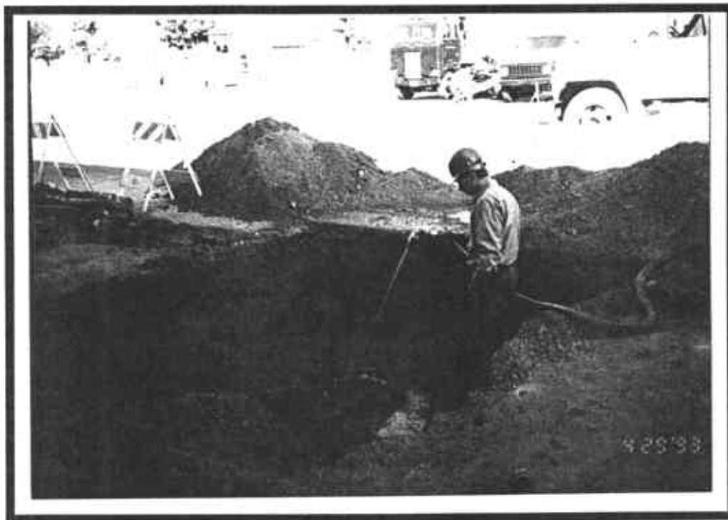
waste oil tank clean-out process
