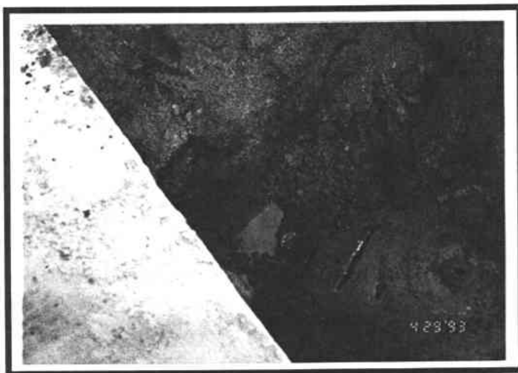
Bulk Oil tank excavation showing deeper groundwater (~11 ft.) and backhoe punctures
