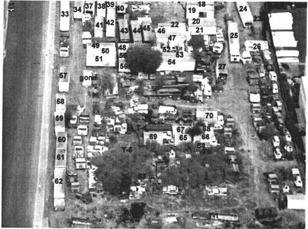
Photo no. 3: Aerial photo looking north with trailers labeled (photo taken on Oct. 3, 2003).
