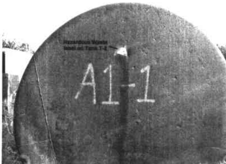
Photo no. 19: Tank T-2 had a worn out Hazardous Waste label on it.
