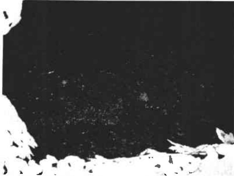
Photo no. 13: The material inside the tank had a thin dark layer of material on the top. This photo was taken through the hole in the tank that is shown in photo no. 11.
