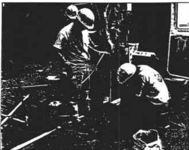
Scott Traub (center) and Volker Wittig (seated) measure out the sand pack which is added above the screened area while setting a Geoprobe Prepacked Monitoring Well.
