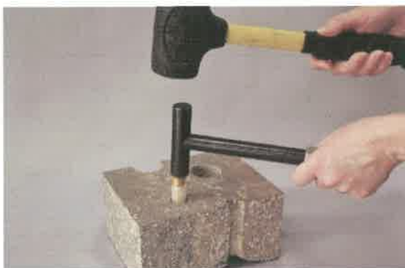
Figure 2. Installing the Vapor Pin™.
