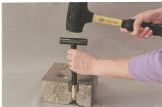
Figure 3. Flush-mount installation.
