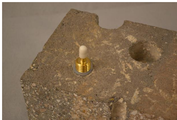
Figure 3. Installed Vapor Pin™
