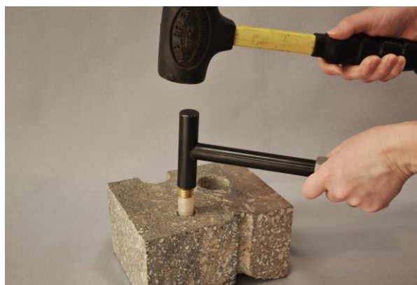
Figure 2. Installing the Vapor Pin™.
