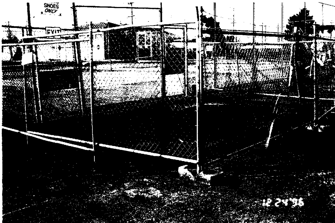
Excavation secured after tank removal
