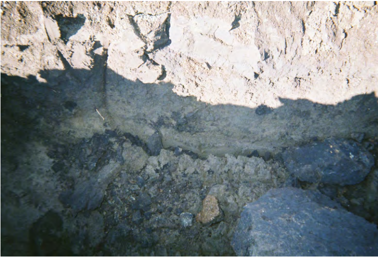
Photos 2 & 3 - View to the west of the north-south trending trench. 0 to 1½ ft bgs is fill composed of vermiculite and ground up bone and red lava rock.
