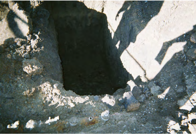
Photo 11 - View to the west of the extended east-west trending trench. See the abandoned water line encountered to the east at the bottom of the photo.
