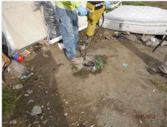
Photo No. 5 - Remove vault box
