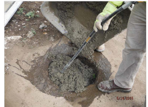
Photo No. 6 - Backfill upper section of borehole with concrete
