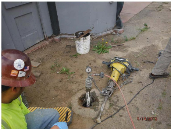
Photo No. 4 - Pressurize grout
