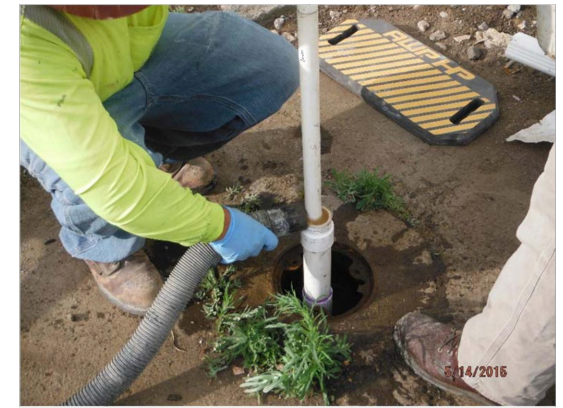
Photo No. 3 - Remove displaced groundwater
