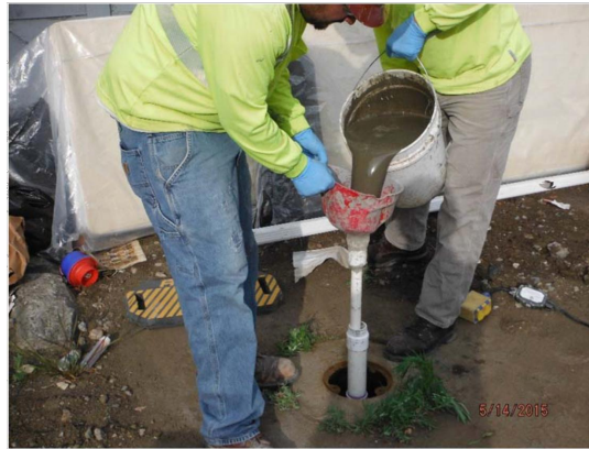
Photo No. 2 - Insert tremie pipe and begin grouting
