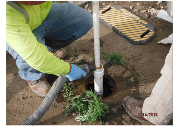
Photo No. 3 - Remove displaced groundwater
