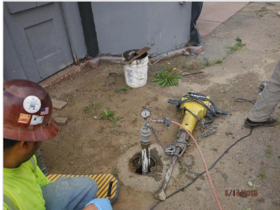
Photo No. 4 - Pressurize grout
