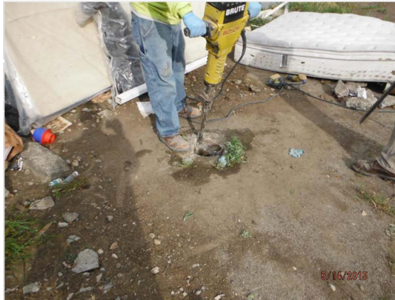
Photo No. 5 - Remove vault box
