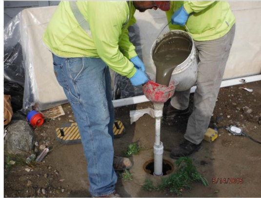
Photo No. 2 - Insert tremie pipe and begin grouting
