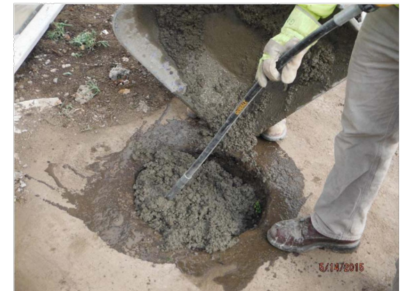
Photo No. 6 - Backfill upper section of borehole with concrete
