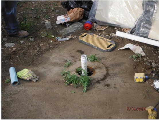
Photo No. 1 - Add PVC adapter to well casing
