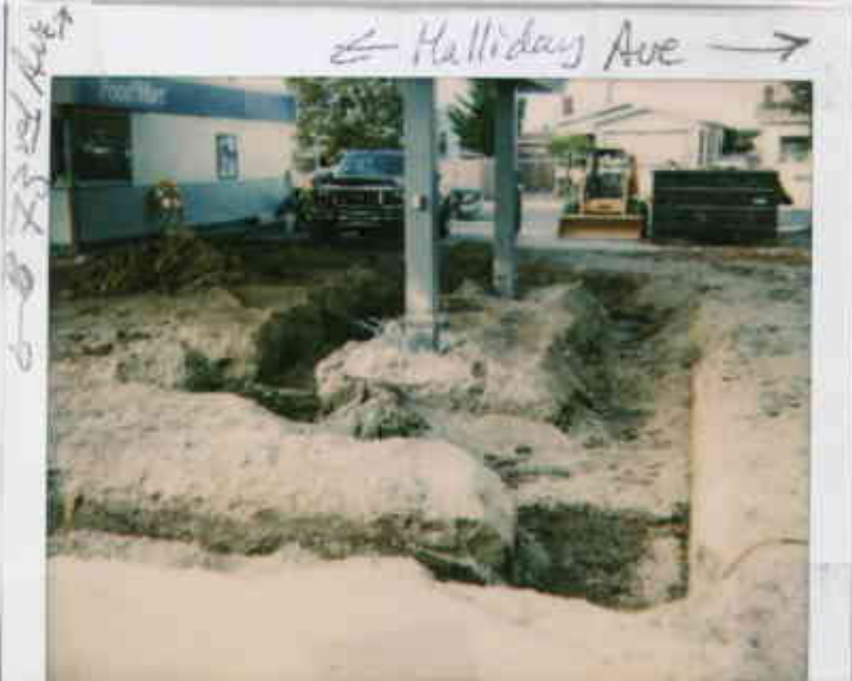
7225 Bancroft Ave, Oakland 8/27/96 05617107379-24 1438 9348 COPIES & ENLARGEMENTS CALL 800-421-1030 Northernmost dispenser & piping & vent line trenches. - Juliet S.
