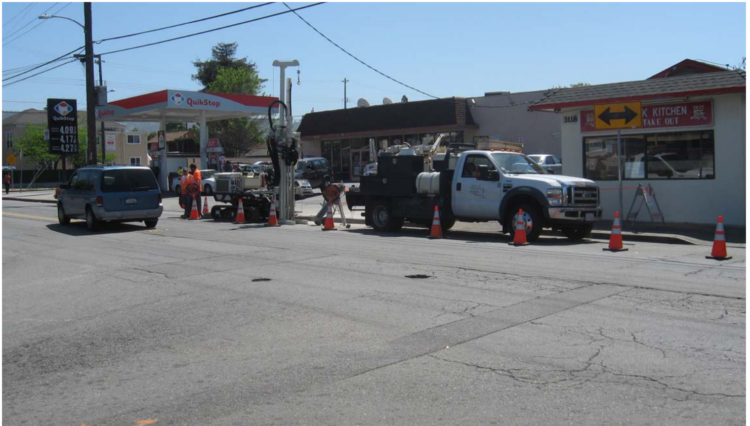
010. Advancing boring DP-3 just downgradient of the active QuikStop fueling facility
