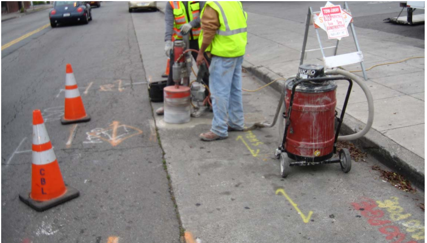
001.Pre-coring concrete at well MW-5 location - avoiding multiple utilities
