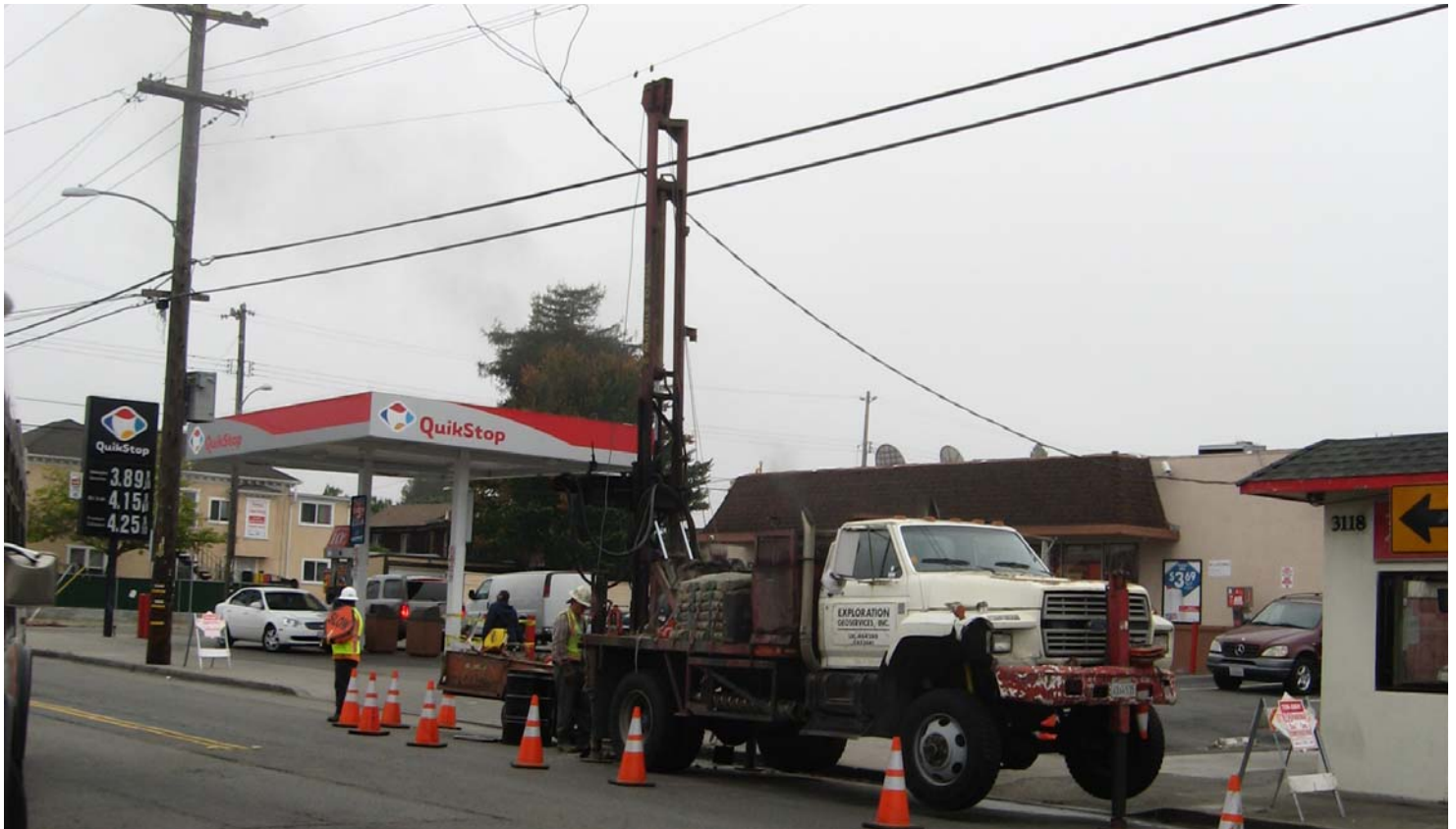
003. Drilling and installing well MW-5
