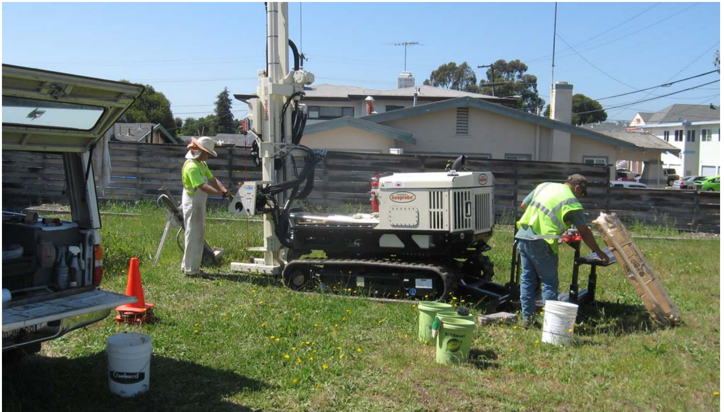
014. On-site drilling and soil sampling
