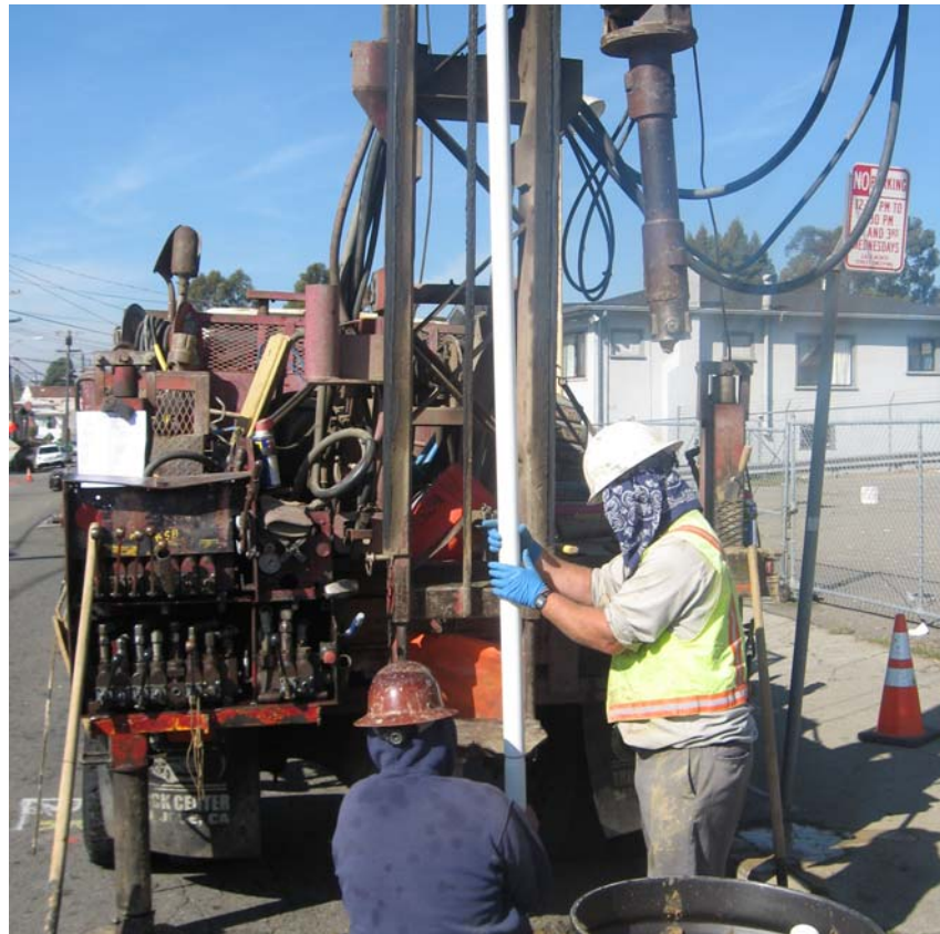
009.Installing MW-6 well casing
