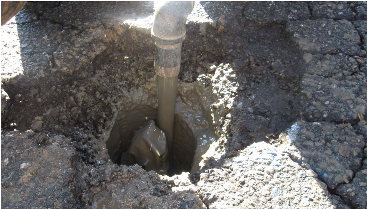
008. Completing well seal at MW-6
