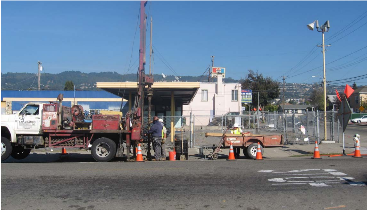
007. Advancing well MW-6
