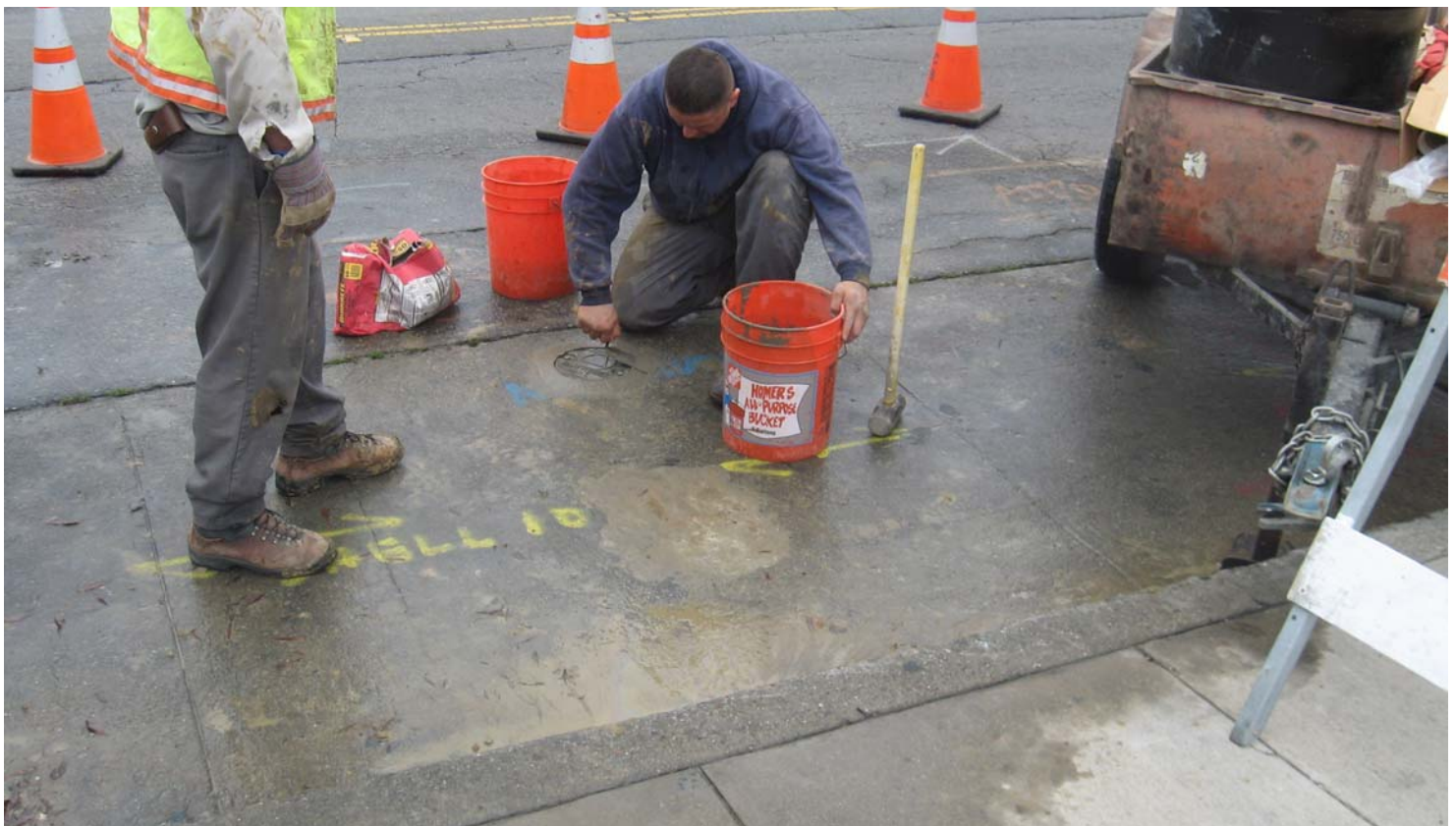
006.Setting traffic rated well box at MW-5
