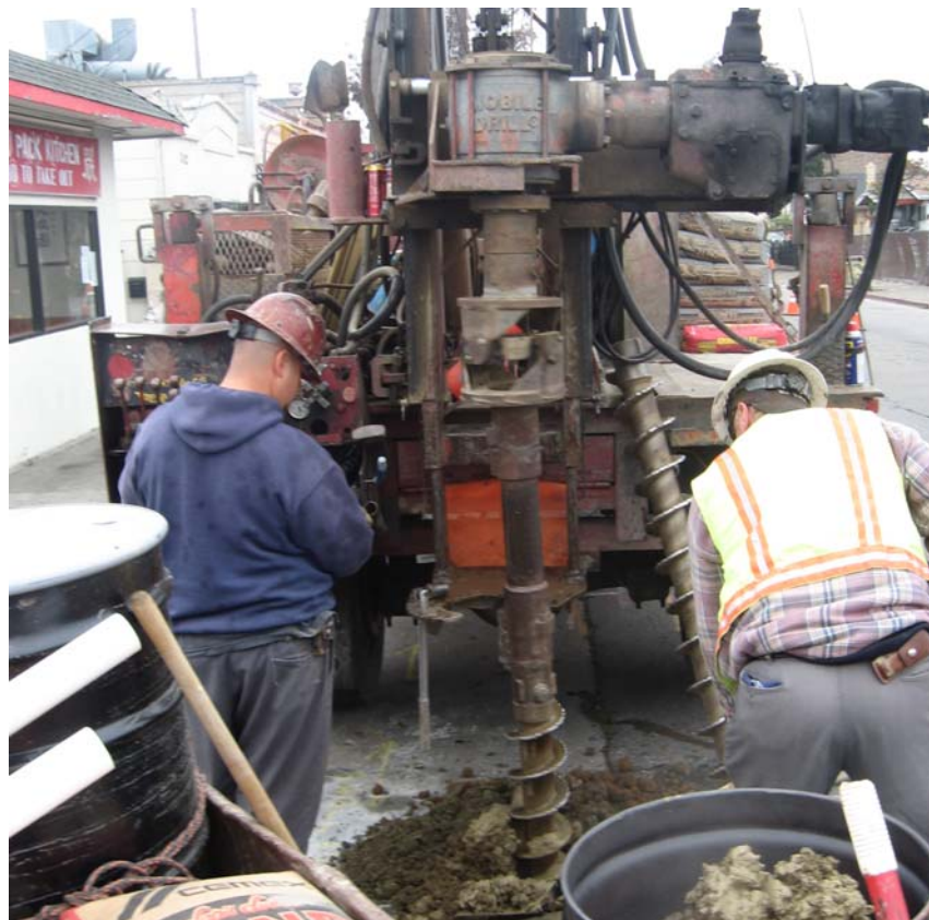
004. Advancing MW-5 borehole
