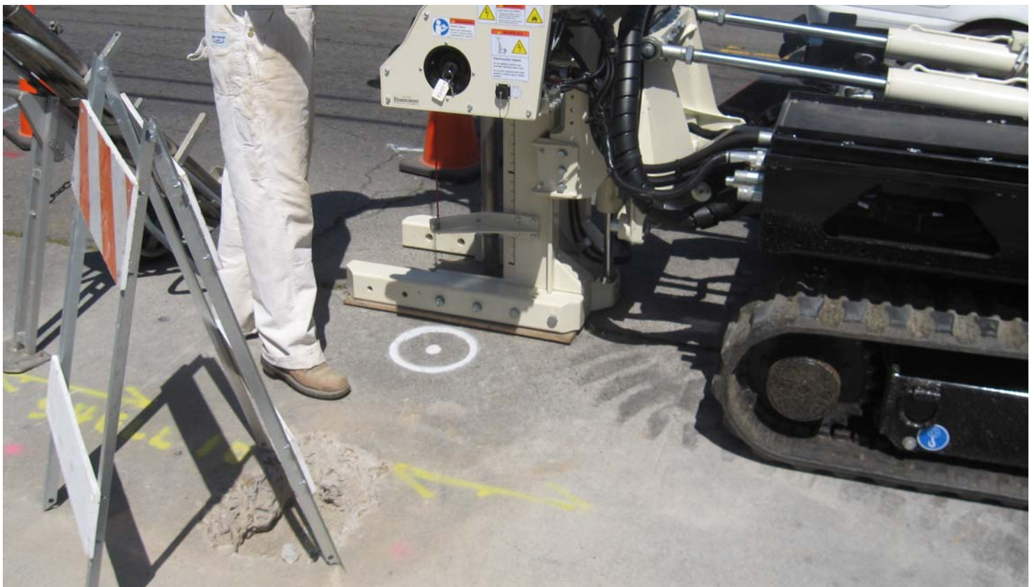
011. Boring DP-3 adjusted to avoid exposed Shell Pipeline
