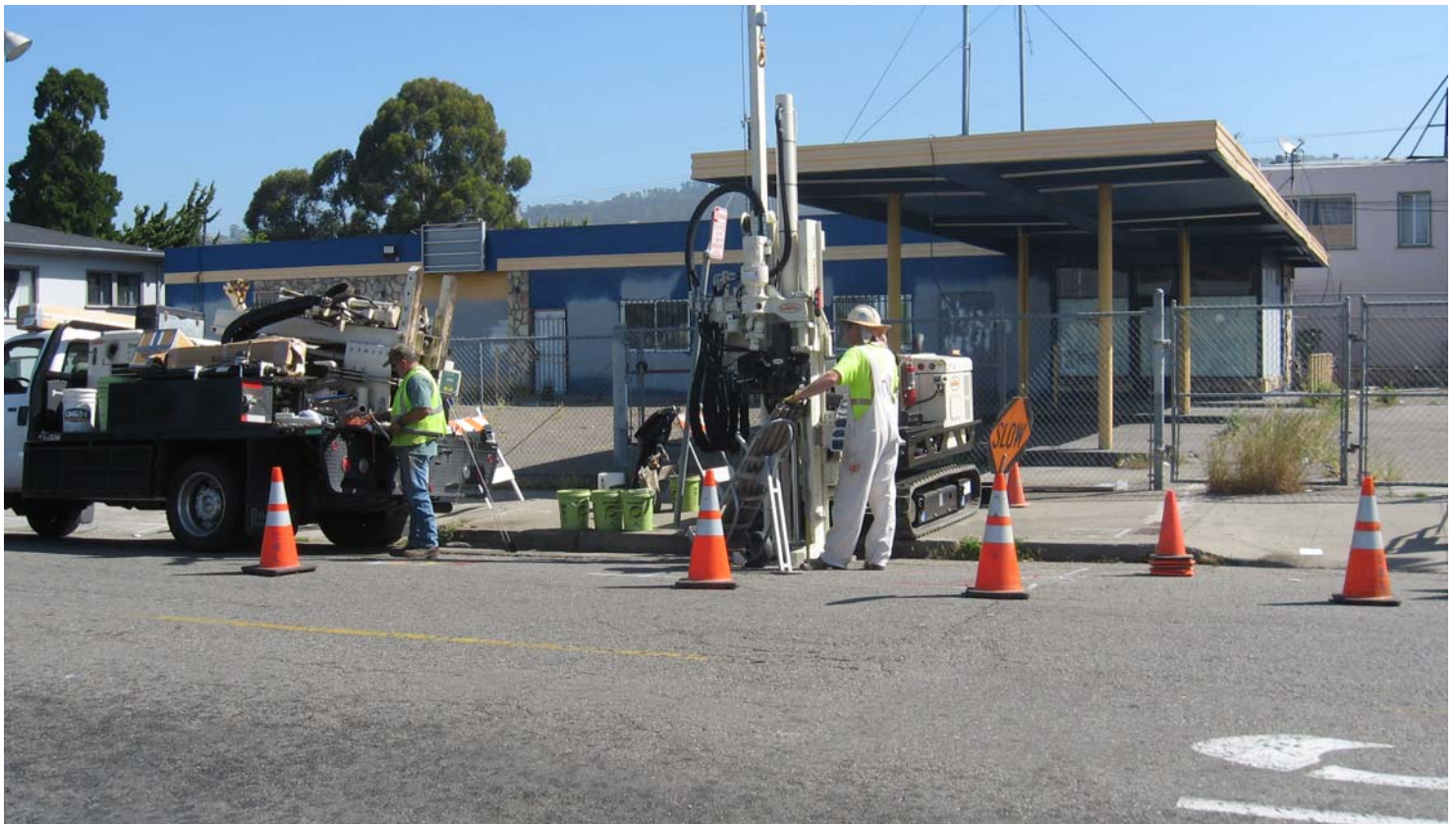
009. Advancing DP-2 just downgradient of abandoned fueling facility
