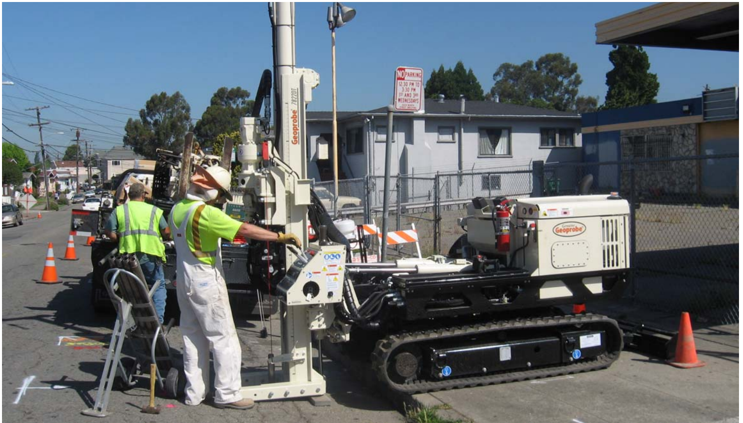
008. Advancing boring DP-2
