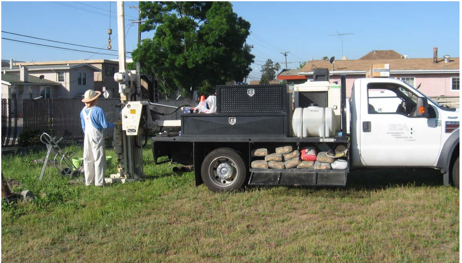
001. Advancing on-site soil borings for soil sampling
