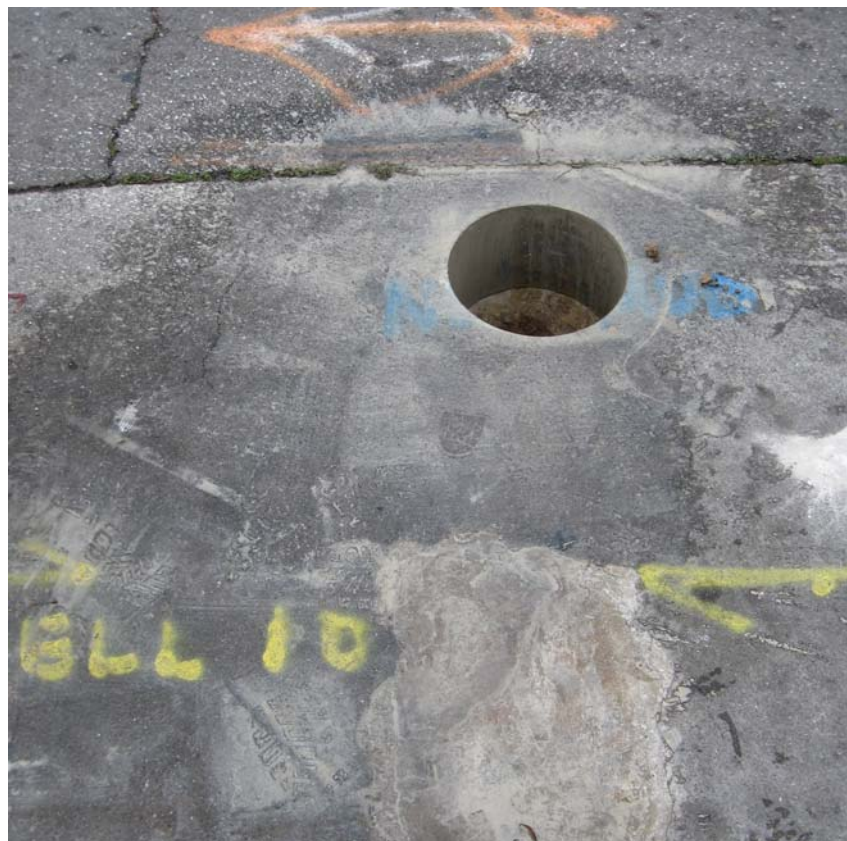
002.Precored concret at MW-5 location
