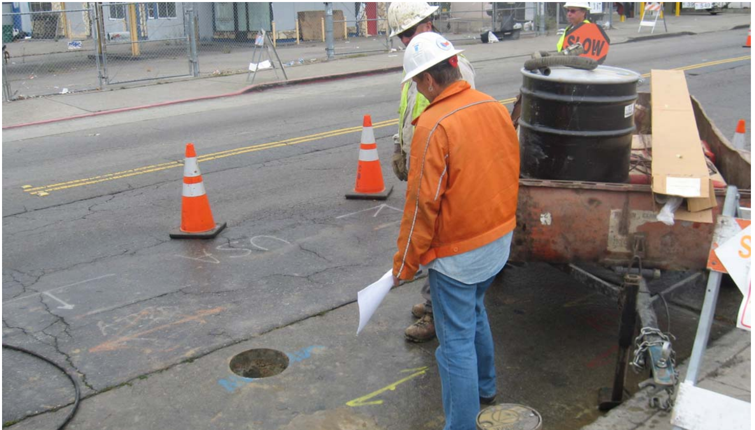
005.ACPW grout seal inspection
