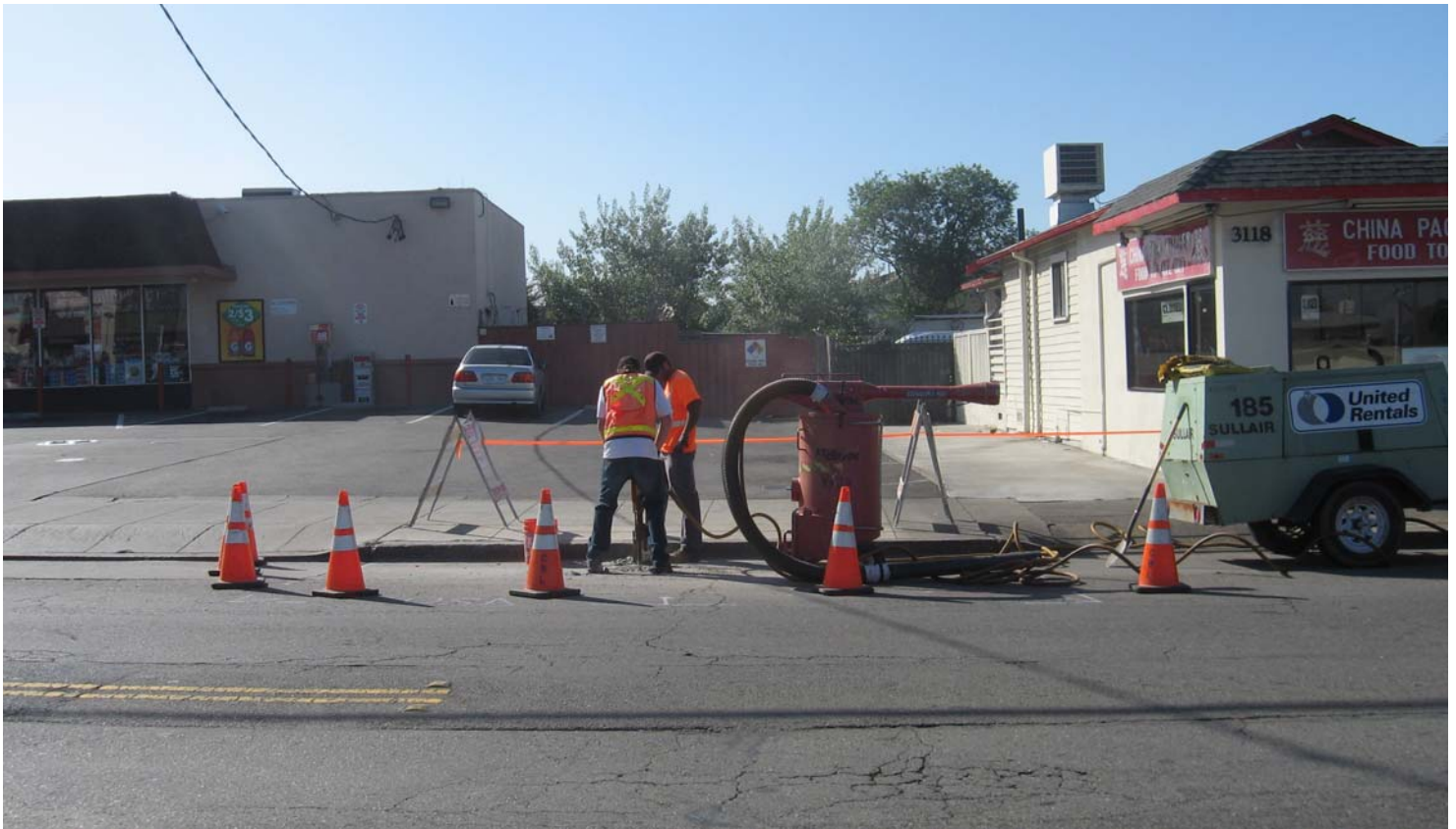
006. Clearing utilities via air-knife at boring DP-3 - required by Shell Pipeline
