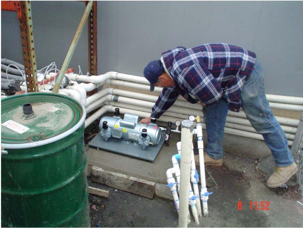
*Install of Air Compressor for Air Sparging*
