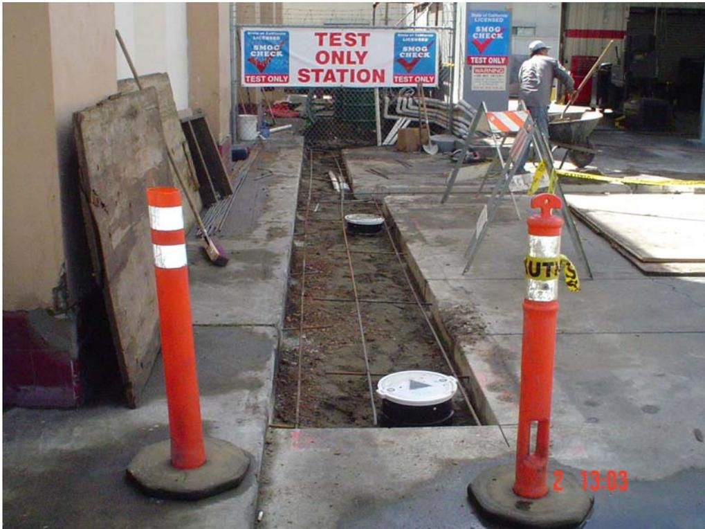
*Rebar Placed in Trench for Concrete Pour*
