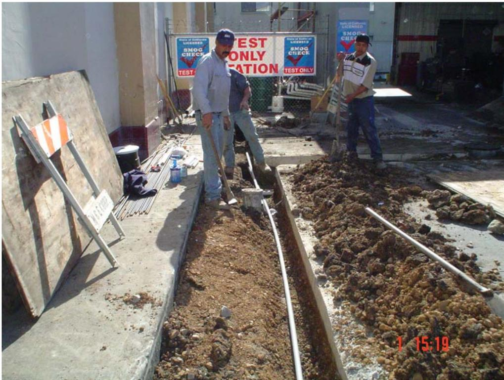
*Install of Piping from Air Sparge Wells AS-4 and AS-5 to Remedial Compound*
