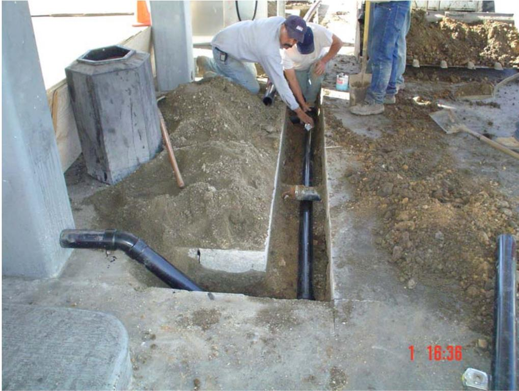
*Install of Drain Line at Down-Spouts of Canopy*
