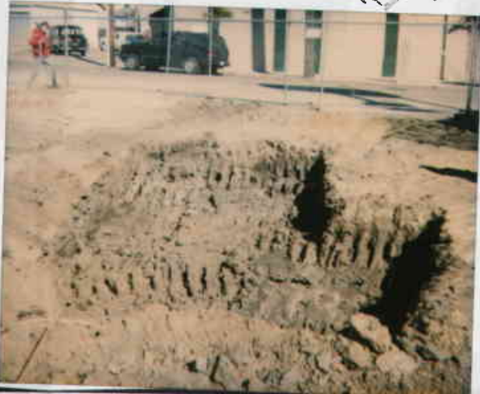
- Juliet Shire 800 San Pablo, Albany 4/11/97 Excavated about 5' deep trench material Surrounding area. ENLARGEMENTS CALL 800-421-1030 Product piping due to strong odors staining
