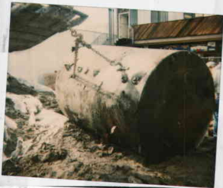
800 San Pablo, Albany 3/5/97 2,000-gallon diesel UST. Older from tank 10617123989-2W 1358 7133 on petrels noted on tank COPIES & ENLARGEMENTS CALL 800-421-1030 Juliet Shinn
