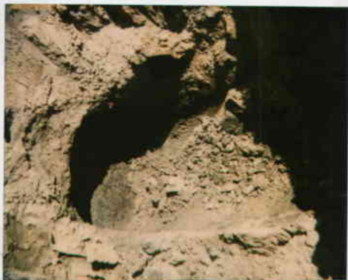
800 San Pablo, Albany 3/31/97 Tank pit of 1,000-gallon gas UST. 1061-123999-24 1357-219 COPIES & ENLARGEMENTS CALL 800-421-1030 - Juliet Shim
