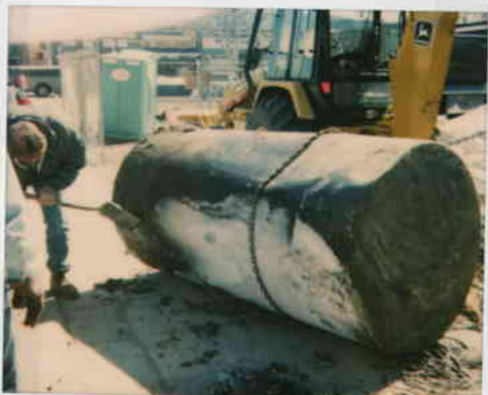
800 San Pablo, Albany 3/31/97 1,000-gallon gas UST. No observed holes. 1061-123999-24 1357-219 COPIES & ENLARGEMENTS CALL 800-421-1030 - Juliet Shim
