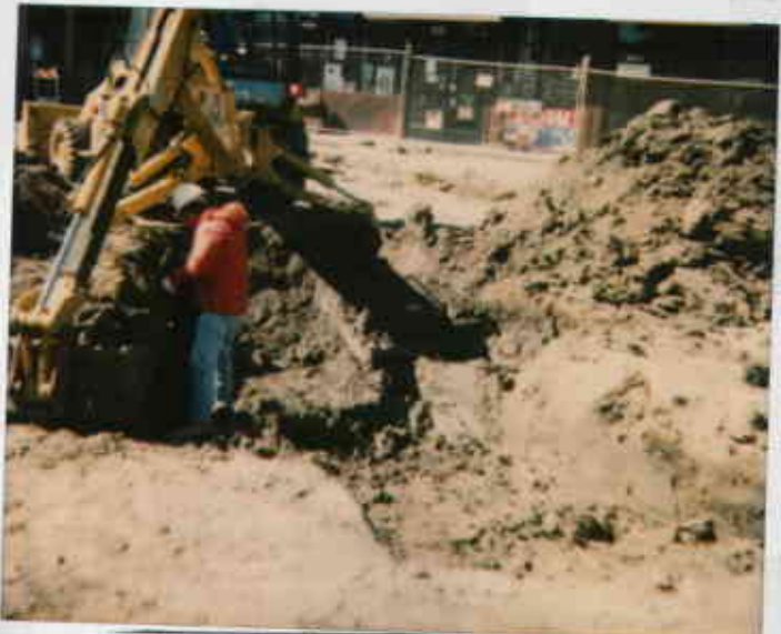
800 San Pablo Albany 4/11/97 Soil samples were collected from below trench material at 2 5' bags. ENLARGEMENTS CALL 800-421-1030 - Juliet Shire
