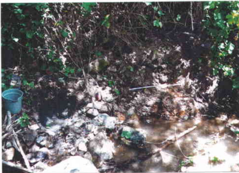
Subject: Borehole HP-11, adjacent to Redwood Creek -- white bailer at right shows top of visibly contaminated soil ("smear zone") Site: Redwood Regional Park Service Yard Fuel Leak Site, Oakland California
