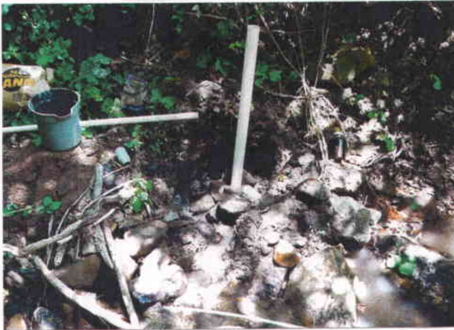
Subject: Temporary well point at HP-11, adjacent to Redwood Creek, prior to damming and purging pit to remove stream water Site: Redwood Regional Park Service Yard Fuel Leak Site, Oakland California
