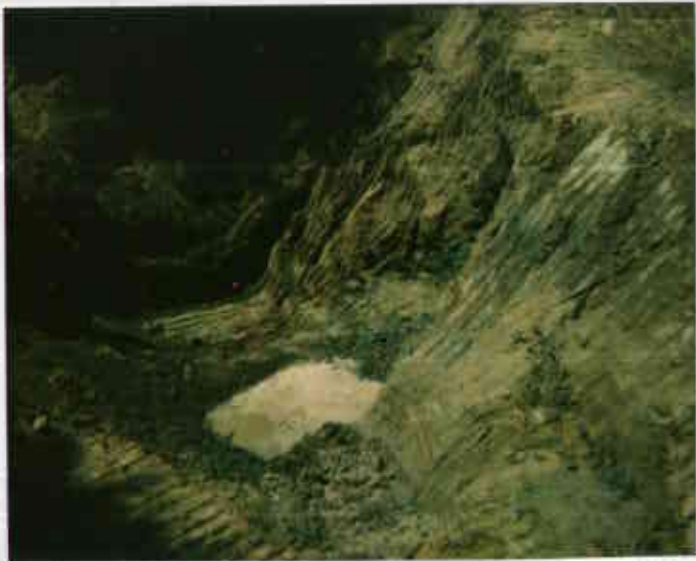
12215117976-8 6/14/93 Redwood Regional Park Overexcavation / Stained Soils Juliet Street 1
