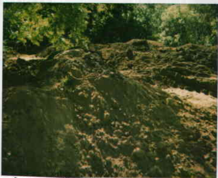
Redwood Regional Park 22215117976-8 6/15/93 Stockpiled soil collected from above tanks. Some contaminated soil accidentally placed in w/ pile. Tuberium 3
