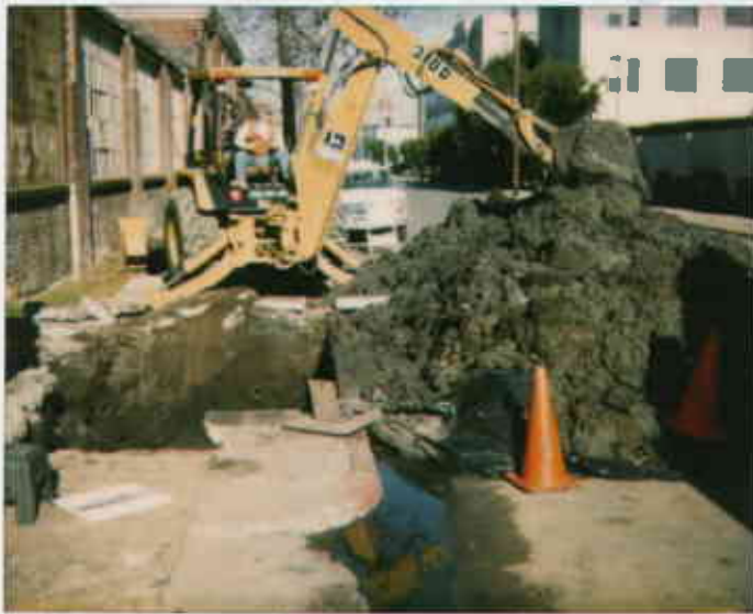
11/6/14 Riflew Pwp - continued access excavation former gas tank
