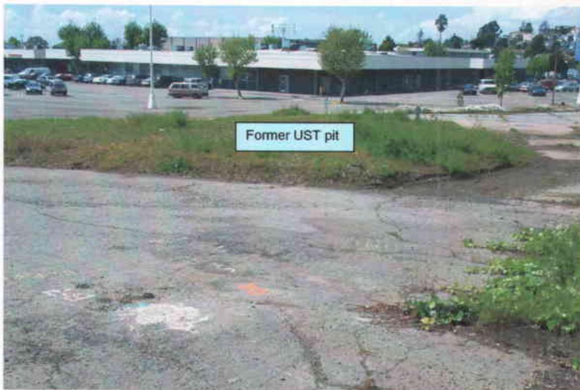
Former UST pit, viewed from 108 th Avenue (facing northwest).
