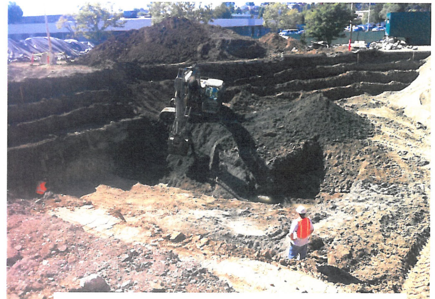
Area of Over-Excavation
