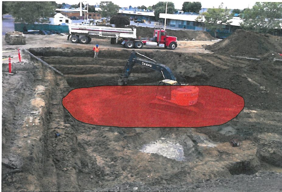
Area of Over-Excavation
