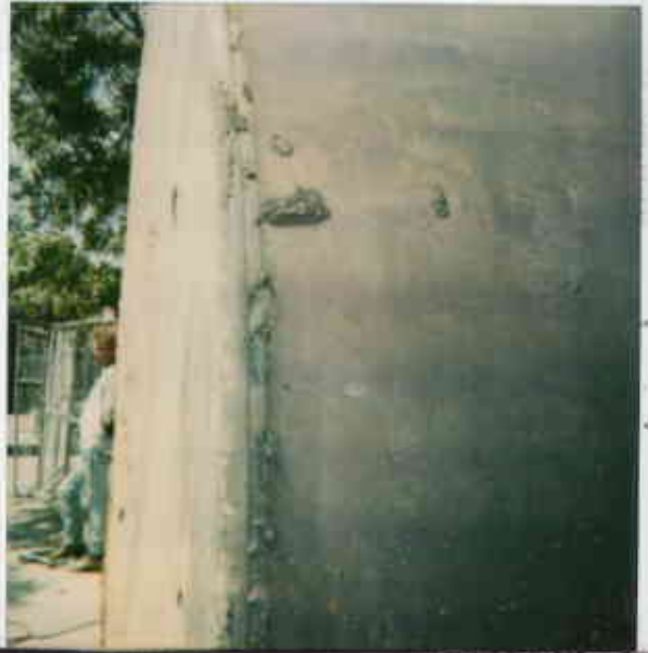
10349032026 POLAROID® 3 10700 MacArthur - Oak 7/19/94 Weld / repair of 12K gasoline UST Tank 3
