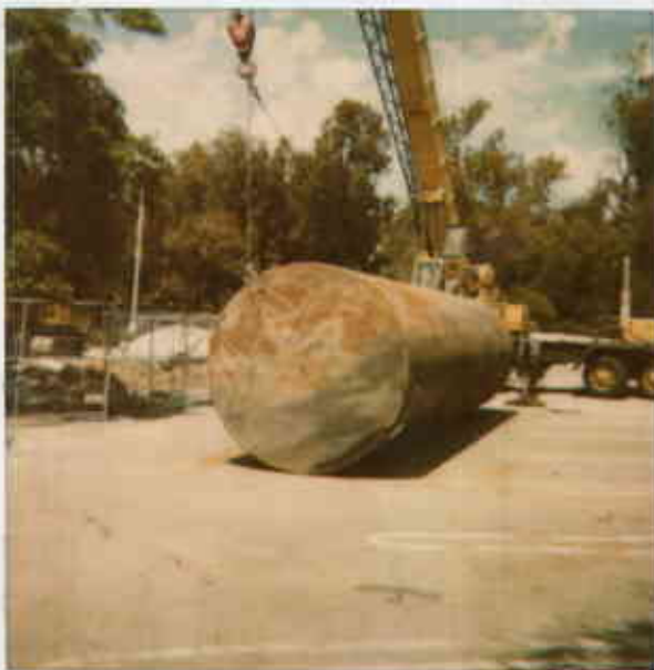
11103127675 POLAROID® 6 10700 MacArthur - Oak 7/19/94 Tank 2 (middle) - 12K USG gasoline Fill end had hole + was leaking water when pulled.
