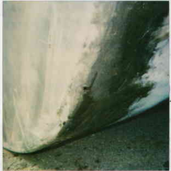
10349032025 POLAROID® 3 10700 MacArthur - Oak 7/19/94 1/2" noted on end segment of Tank 1 - (12 Keys)
