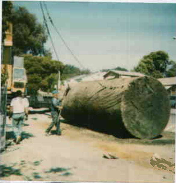
10349032028 POLAROID® 3 10700 MacArthur - Oak 7/19/94 8K tar wrapped diesel UST Tank 4
