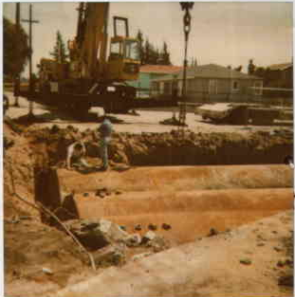
11103127675 POLAROID® 6 10700 MacArthur - Oak 7/19/94 3 gasoline USTs (12 Each) in pit Tank 4
