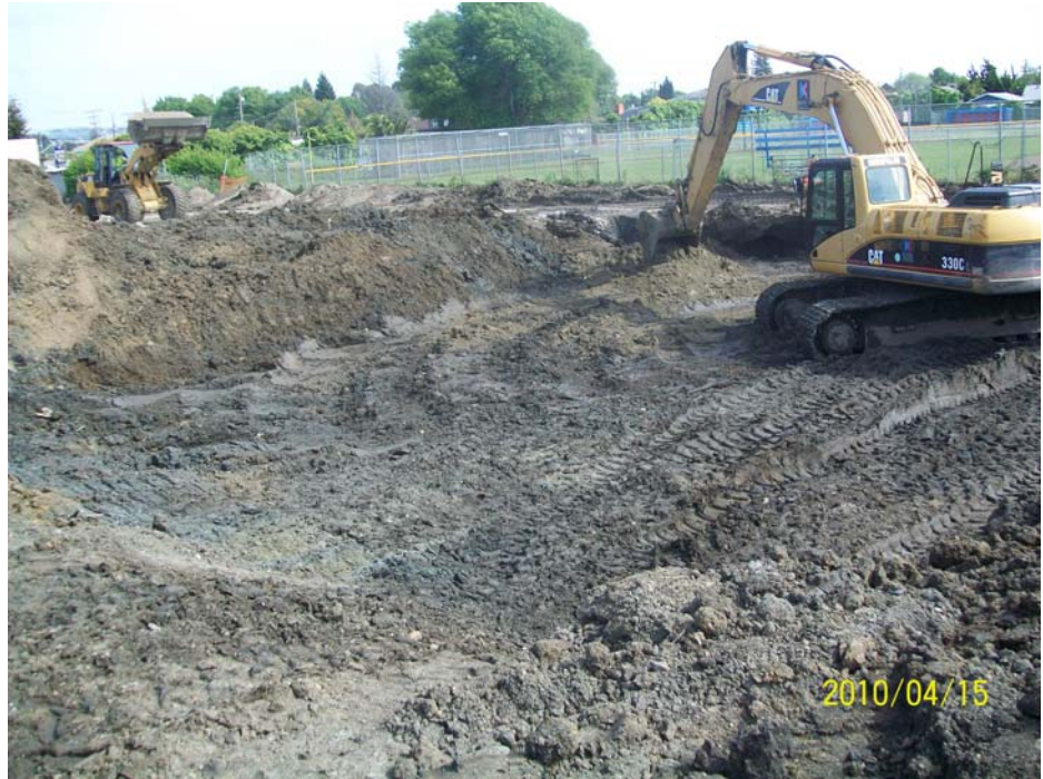
View of soil backfill within re-excitation, facing southeast
