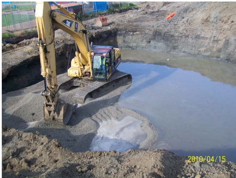
View of rock placement within re-excavation, facing southwest
