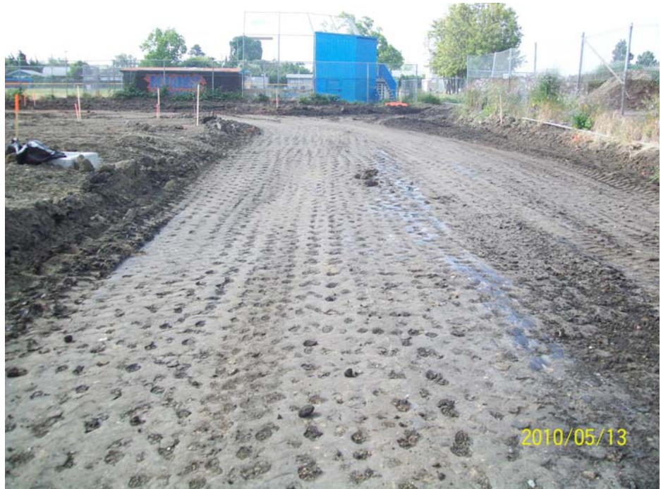
View of compacted roadway subgrade, facing south
