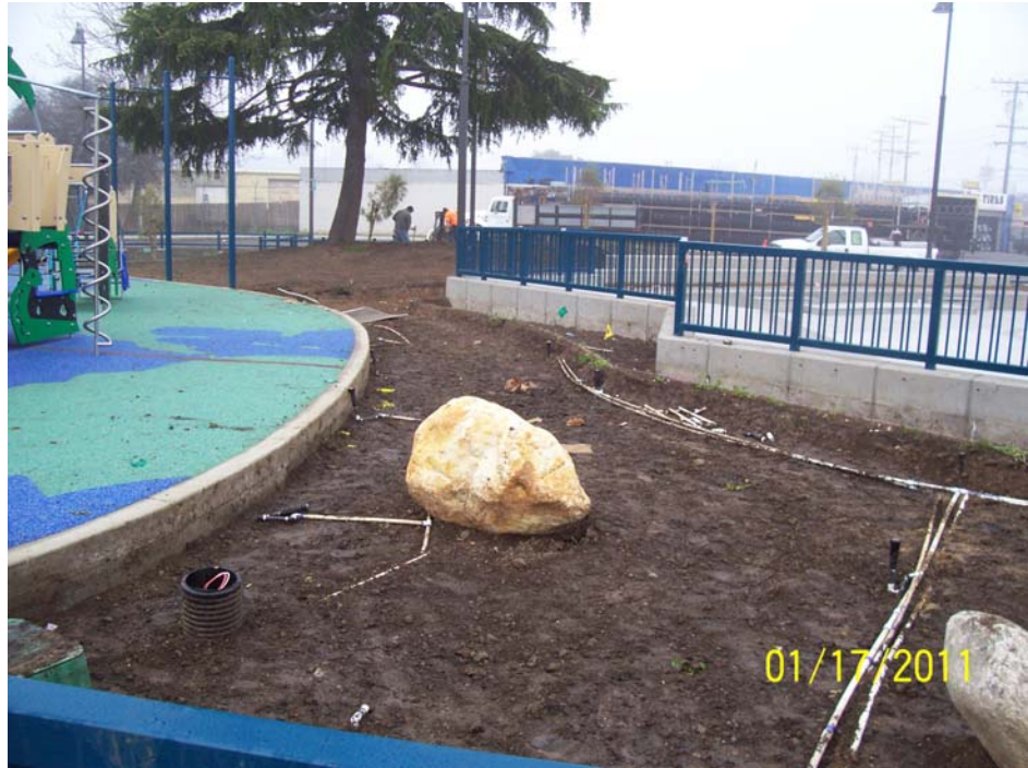
View of soil subgrade after re-excitation between play area and skate-park, facing west
