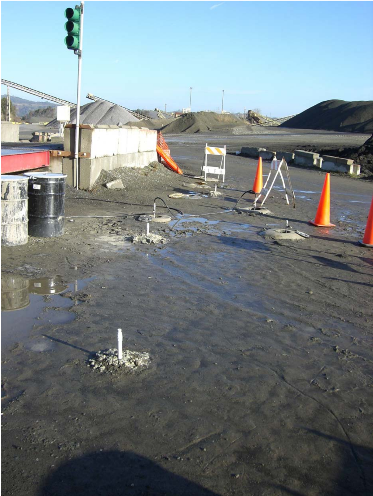
Photograph 4: Soil-Gas Sampling Points and Air Sparging Wellheads Surrounded by Puddles.
