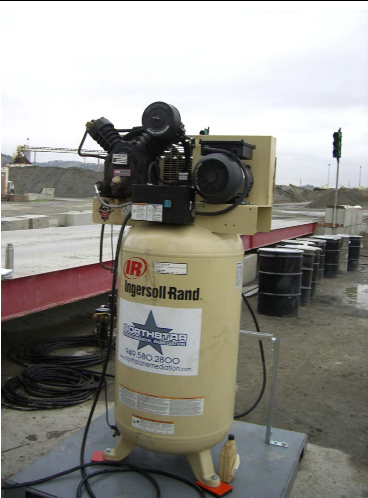
Photograph 1: Air Sparge Pilot Test Compressor.
