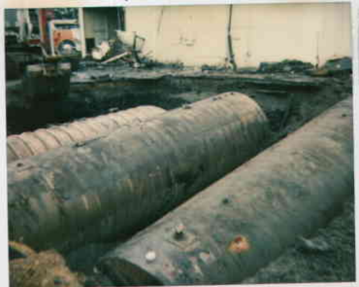
3-10K tanks in pit @ 566 Heg Rd. 12/17/92
