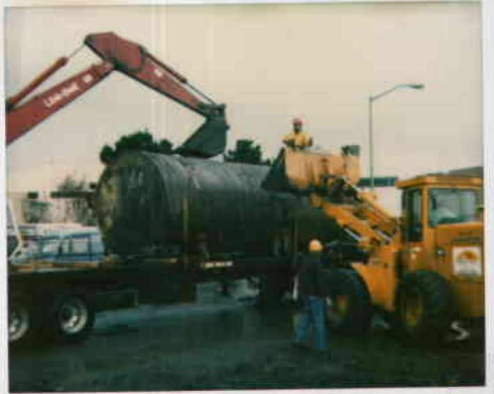
Middle Street tanks, some wrap 566 Heg 12/17/92 deteriorated
