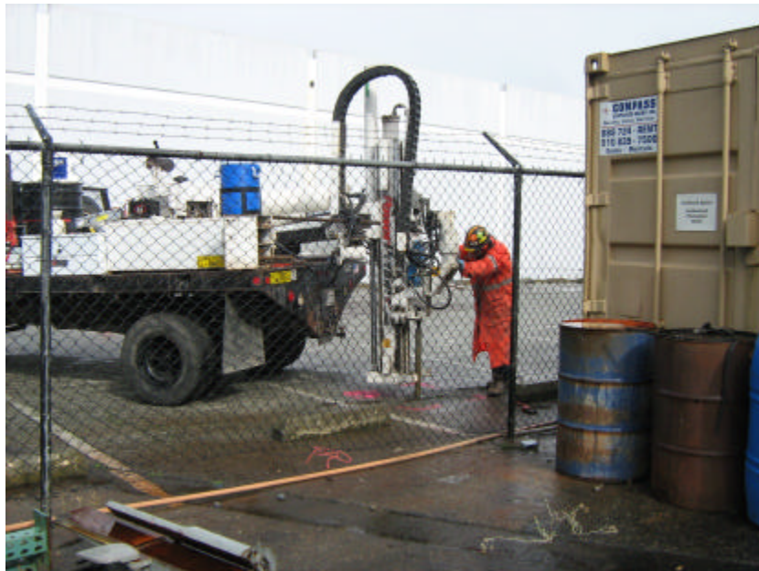
Photograph 2 – View of the drilling rig equipped with direct push technology (DPT) advancing boring TR-4)
