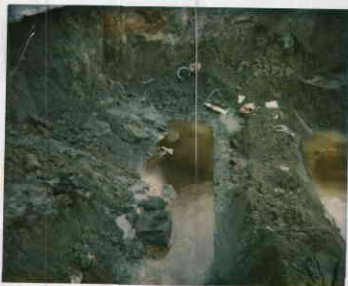
1701 Park St, Alameda 4/8/84 Floating product over water in pit of four 10,000-gallon USTs at site. 09318221467-2 JULIET SLUIJ
