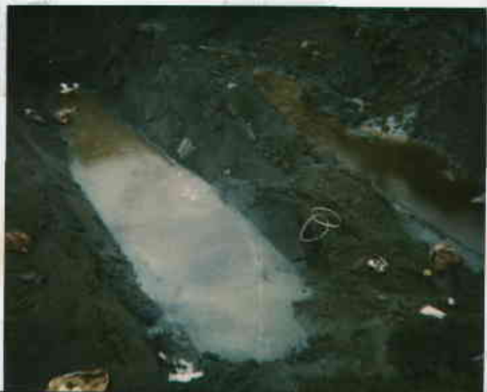
1701 Park St, Alameda 4/8/84 Floating product on water in pit of four 10,000-gallon USTs at site. 09318221467-2 JULIET SLUIJ
