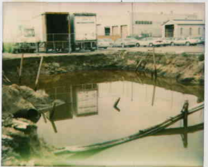
3-29-92 Main tank pit Giberle ANR Freight 2225-7th St, Oakland CA
