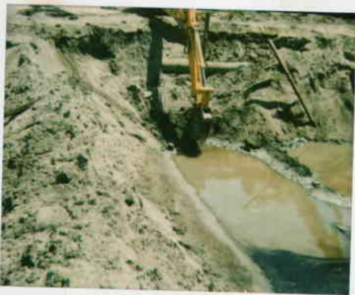
Point 3 (at 25000 gal) Sample location ANR Freight, 2225 7th St
