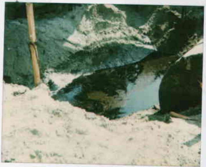
Pit #1 tanks 1 & 2 2225 7th St, ANR Freight 7-27-92
