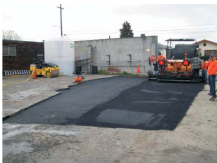
Photo 15. Placing second lift of AC.
