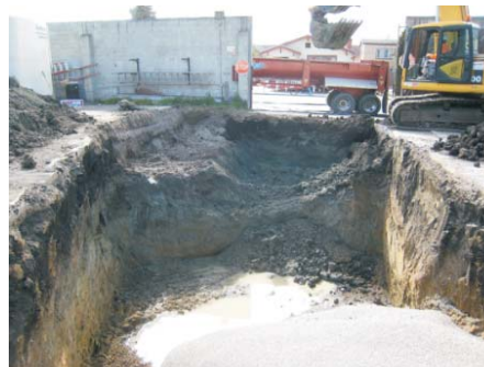
Photo 6. Encountering shallow soil impacts at south end of excavation.
