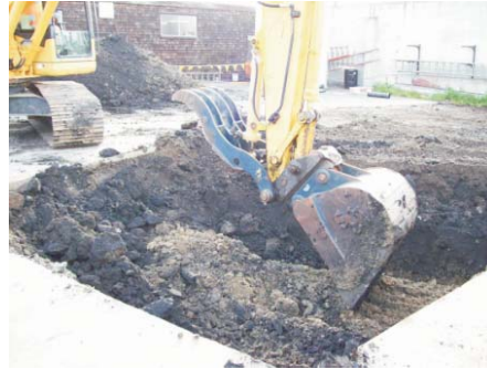
Photo 2. Beginning of soil excavation.
