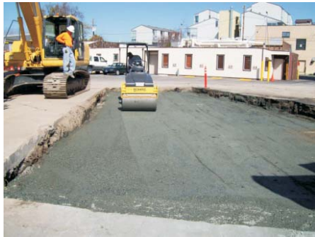
Photo 11. Compacting Class II base rock.
