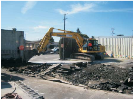
Photo 1. Taking up and removing asphalt.
