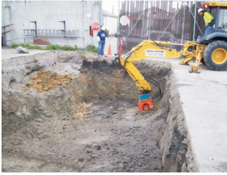
Photo 9. Compacting fill with vibratory equipment.
