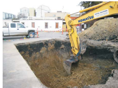
Photo 4. Excavation moving north to south.
