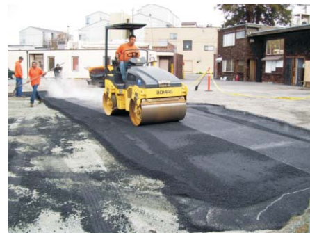
Photo 14. Compacting AC pavement using drum roller.
