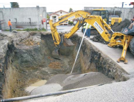
Photo 7. Soil excavation with de-watering sump.
