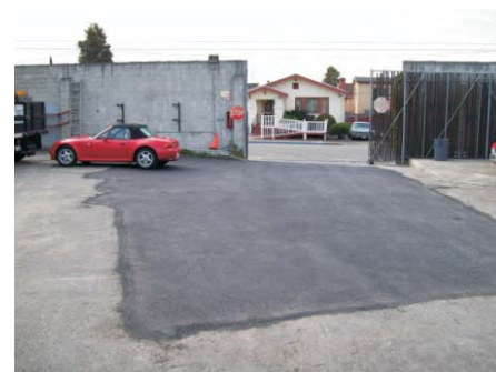
Photo 16. Completed resurfacing of excavation area.
