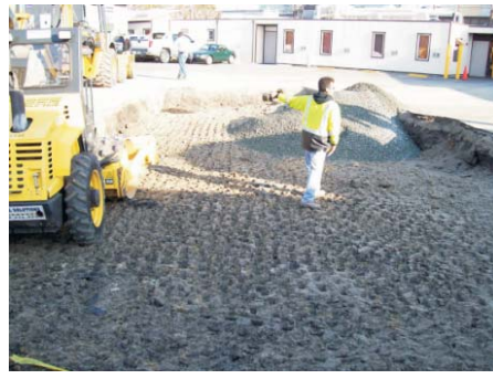
Photo 10. Compacting of fill with "pad" drum.
