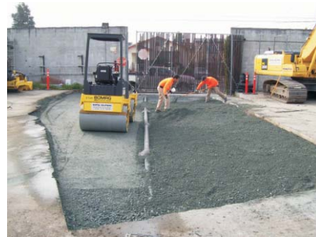
Photo 12. Placing and compacting base rock next to repaired drain line.
