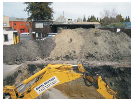
Photo 8. Soil stockpile on east side of excavation.
