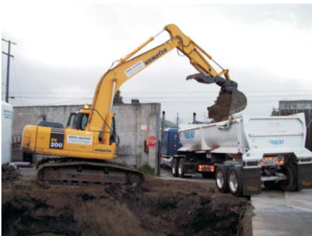
Photo 5. Loading soil into end dump truck.
