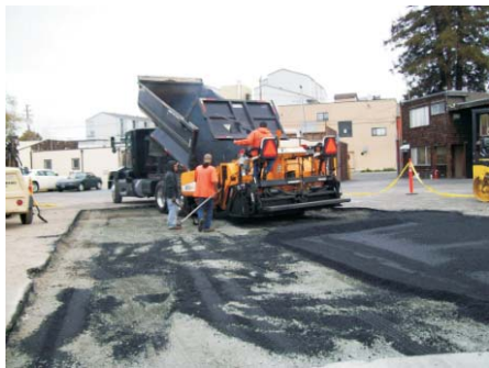
Photo 13. Placing first lift of AC pavement.
