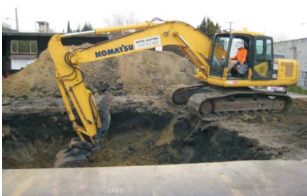
Photo 3. Excavating and stockpiling soil.
