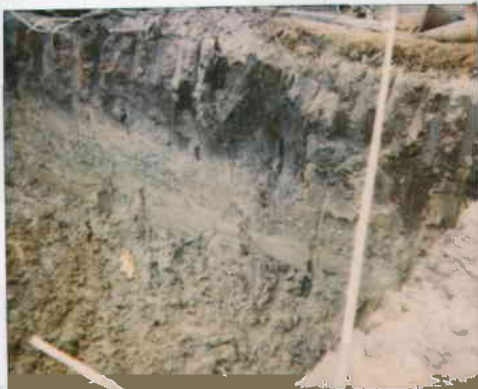
10/25/96 ST 103314 04618111090-24 1348 7856 COPIES & ENLARGEMENTS CALL 800-421-1030 Over site - hot area + dispenser cabinet to avoid weather
