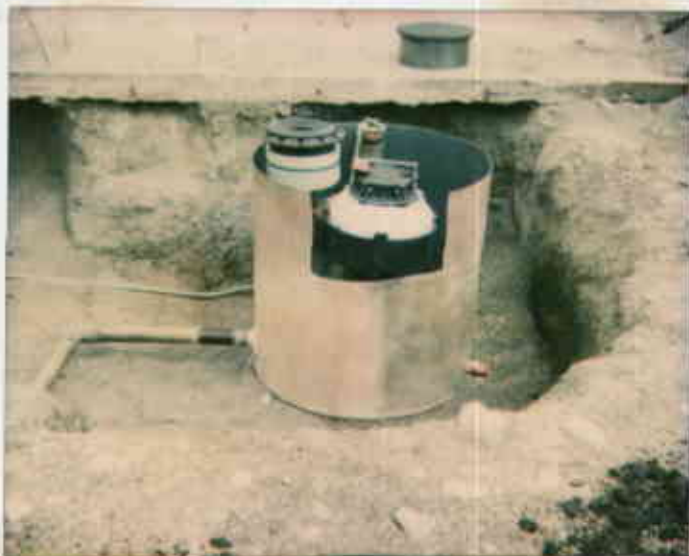
7/6/93-Photo taken by Ron O'Carroll at Bansal shell, 2120 Montana Ave, Oak. Shown is new sump that failed sump test twice. Also note oil cont. of side wall adjacent to it. @
