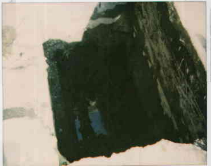
Looking down into well/pit w/ GW apparent 7/28/94 2417 Broadway
