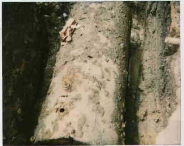
~ 500-gallon gasoline tank 2417 Broadway holes apparent on top
