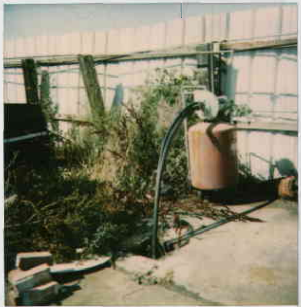
3744 Depot Rd Hayward 8/29/95 On-site domestic well located approx west of waste oil tank
