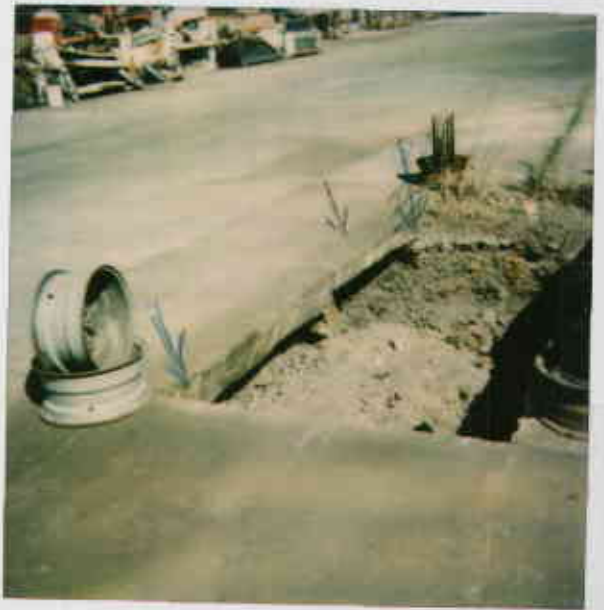
3744 Depot Rd. Hayward 8/29/95 Location of soil borings collected from waste oil tank pit
