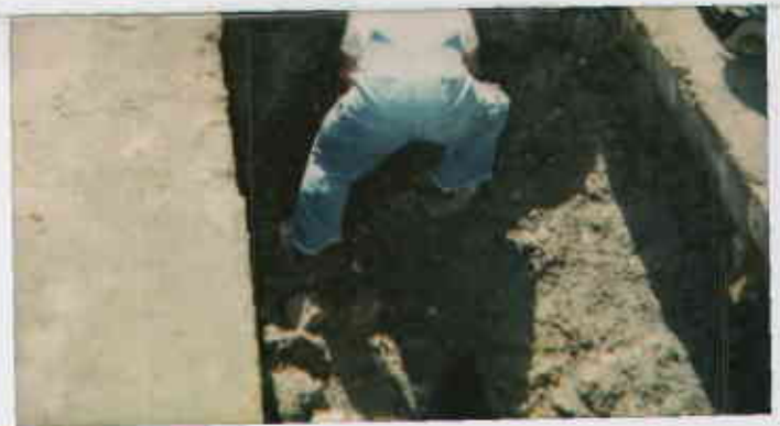
waste oil tank pit 9/30/94
