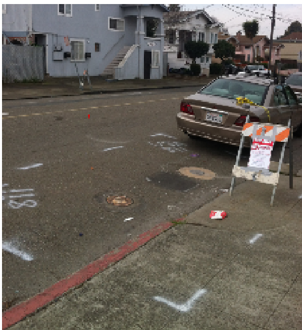
5 January 2012. View of wells MW2 and MW4 before decommissioning/abandonment.
