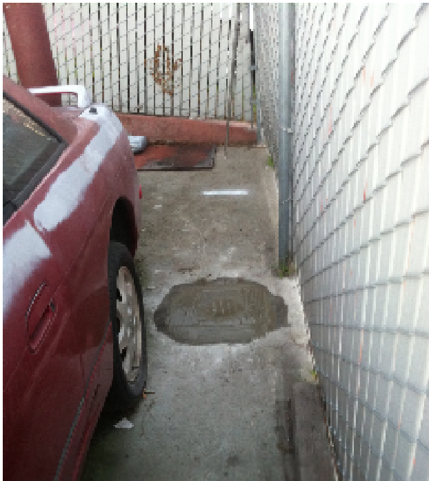
5 January 2012. View of well MW3 after decommissioning/abandonment and subsequent pavement repair. The well-head vault was not removed.
