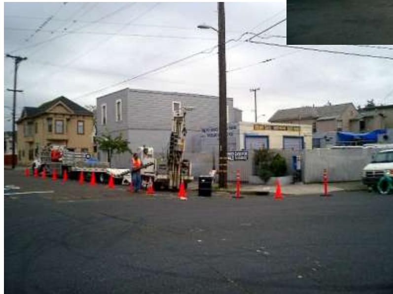
Photograph No. 3 - view southeast of subject property from intersection of 16 th Street and Peralta Street. Auto repair building at center of photo with church and residences behind. Photo shows drilling of exploratory borings within 16 th Street.
