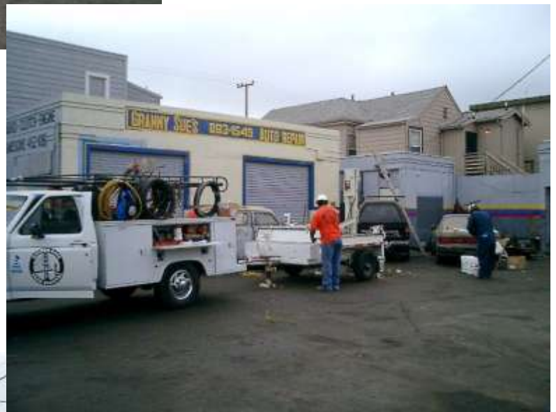
Photograph No. 2 - view of two-bay vehicle repair building and small storage building operated by Granny Sue's Auto Repair. Residence on adjoining property to south. Preparing for drilling activities on August 21, 2008.
