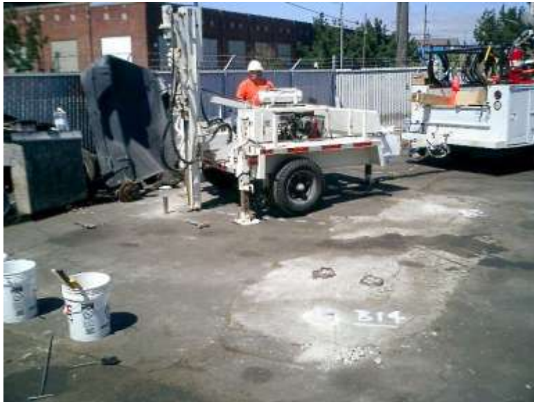
Photograph No. 5 - view northeast of vacant lot at northeast corner of 16 th Street and Peralta Street – former McKinney Service gasoline station. Residence shown on right side of photo and commercial building in background. Drilling and installation of monitor well MW-9 in sidewalk of 16 th Street.
