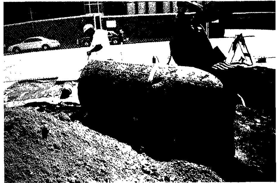
Photo 2: UST after removal.
