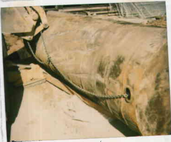
10-12-94 DWESTON STID 3335 TOP OF STEEL TANK (ZINC COATED)
