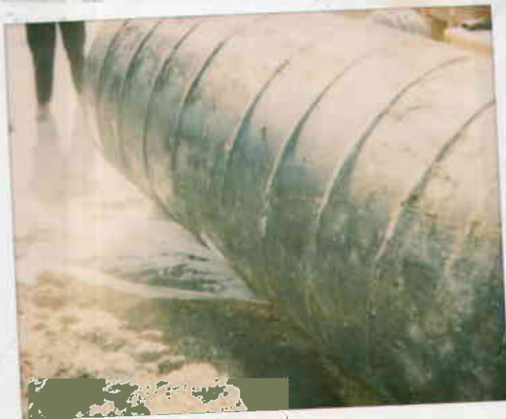
10-12-94 DWESTON STID 3335 SOME CORROSION TANK INTERIOR - NO OBVIOUS HOLES
