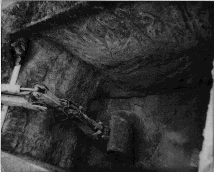
1/11/94 west looking east 1234 40 th Ave gas pit
