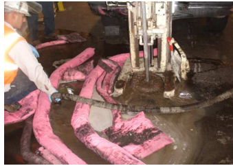
Vironex crew member controls day lighting with a vacuum and socks.
