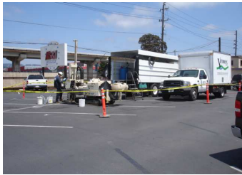
EOS injection in the parking lot area.
