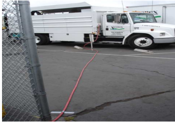
Water for mixing and injection was provided from onsite hose bibs
