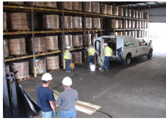
RegenOx/ORC-A injections inside the warehouse area.
