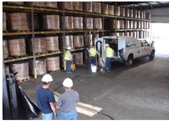
RegenOx/ORC-A injections inside the warehouse area.
