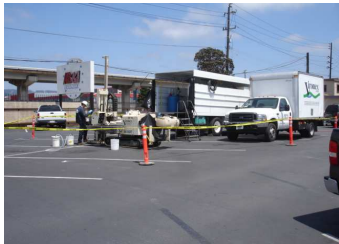
EOS injection in the parking lot area.
