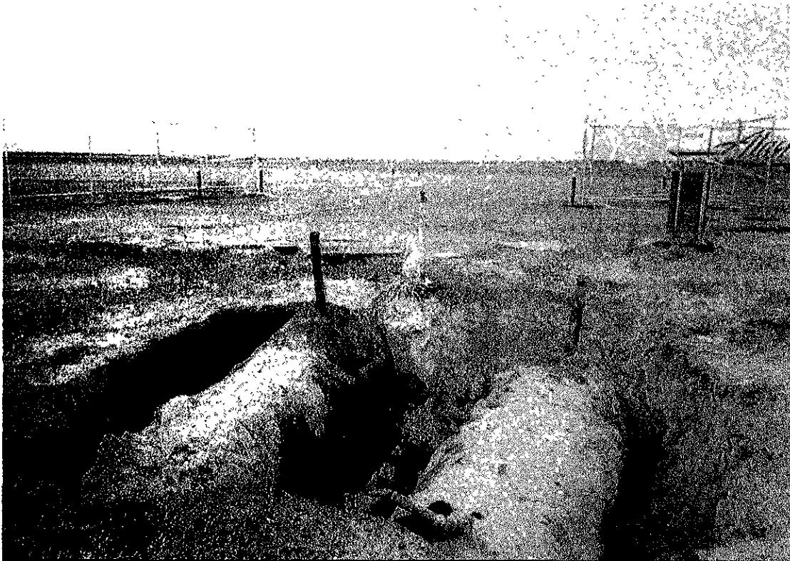
MF9 & MF10, Diesel USTs
