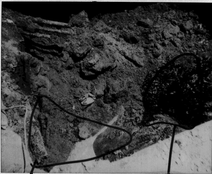
sludge which leaked from UST
