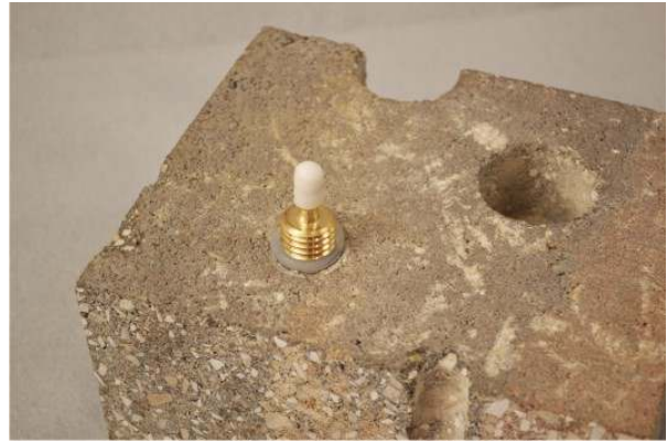
Figure 4. Installed Vapor Pin™.
